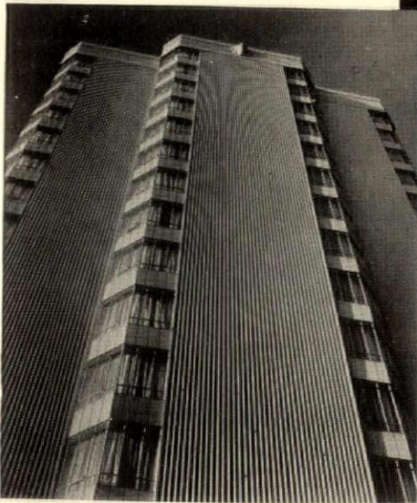
★ No other material is so ideally suited to modern design. Here is a facade, executed entirely in monolithic concrete, on the Edmond Meany Hotel in Seattle, Washington. Architect: R. C. Reamer. Contractors: Teufel & Carlson.
