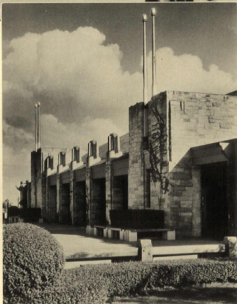
The north building of the East Bath House, which houses the managerial offices, ticket booths, suit-and-towel counter, key counter, and a depository for valuables. The finials of the piers between the towers are lighting fixtures
