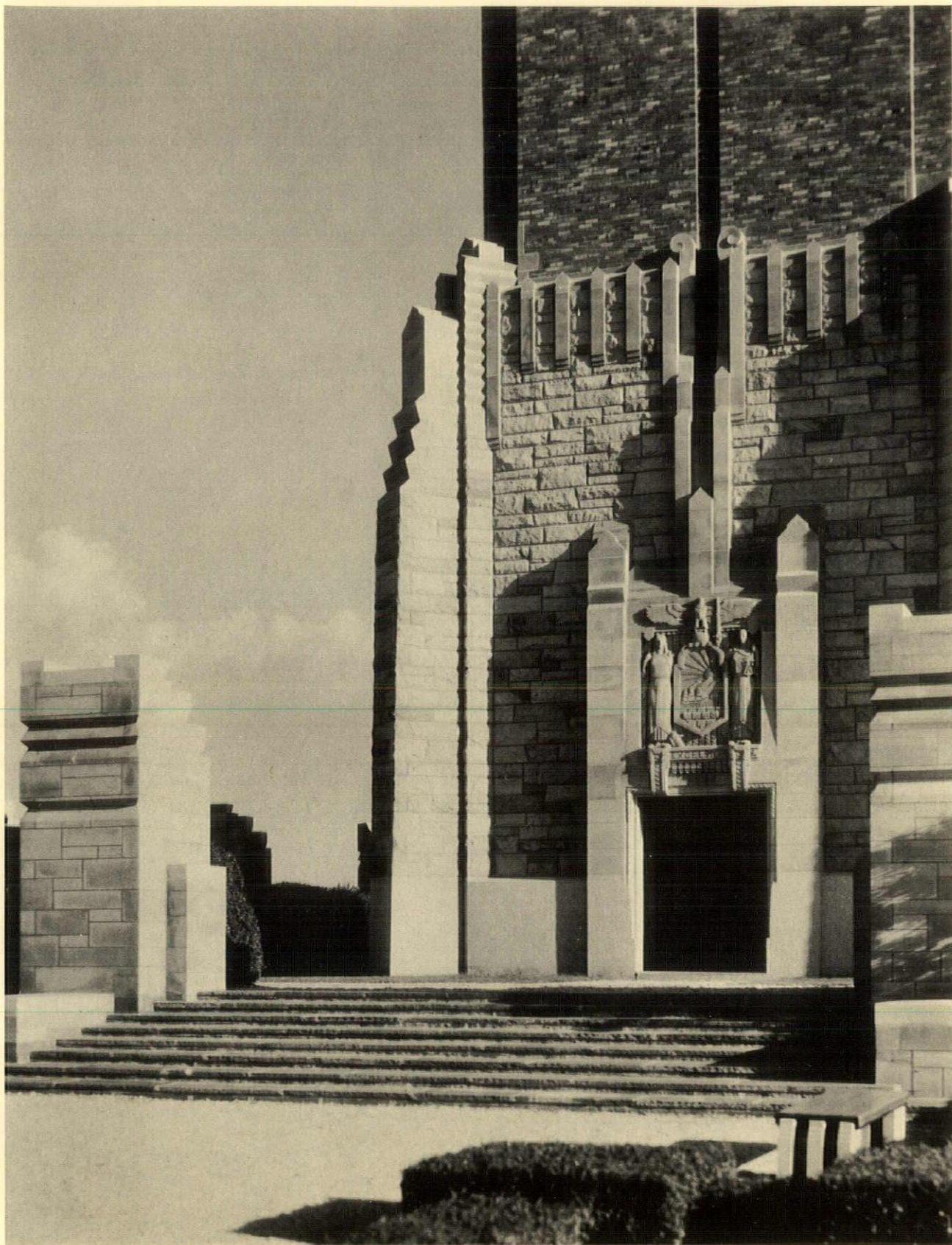
Sandstone is used for the base of the tower, trimmed with limestone. The piers, of which two are shown at left and right, contain the concealed lighting which illuminates the tower at night
