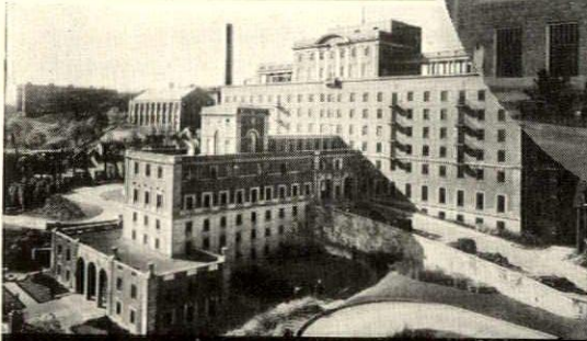
● Montefiore Hospital, Pittsburgh — Henry Hornbostel, Consulting Architect. Genuine Wrought Iron specified for main supply, cold water lines 2" and larger, all waste lines, vents and drains; heating supply lines; exposed radiator returns and special vacuum lines; refrigeration brine lines; high pressure and intermediate steam lines; and compressed air lines.
