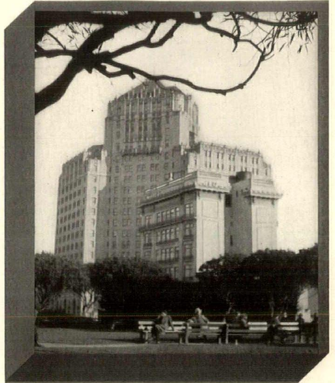
MARK HOPKINS HOTEL, SAN FRANCISCO WEEKS & DAY, SAN FRANCISCO, ARCHITECTS McDONALD & KAHN, SAN FRANCISCO, GEN'L CONTR'S CALKED BY PARKER WEATHERSTRIP CO., SAN FRANCISCO
