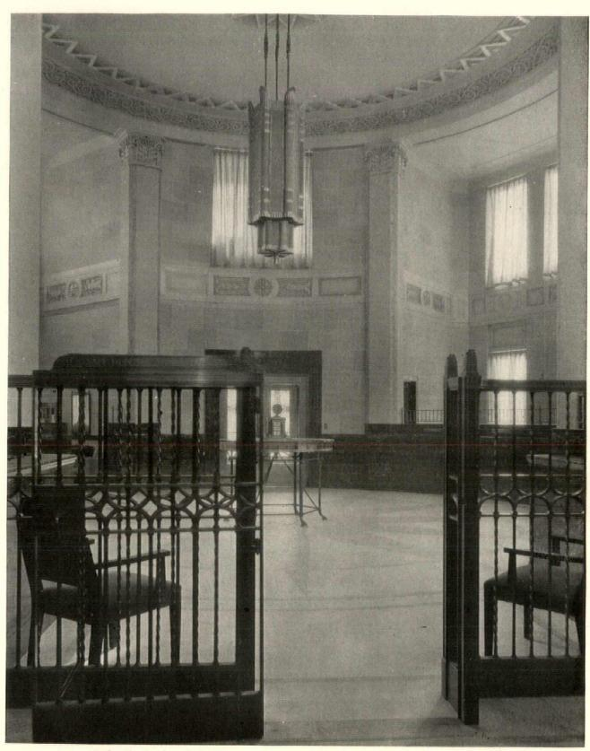
As finally developed, the hexagonal form of the banking-room is cut by the entrance segment, without, however, detracting unduly from the original scheme. The ceiling here is twenty-three feet high, lighted and ventilated on all six wall surfaces by windows in the upper portion leading directly to the outside air and light. The gene al color scheme of the room is that of Caen stone with decorations in old ivory
