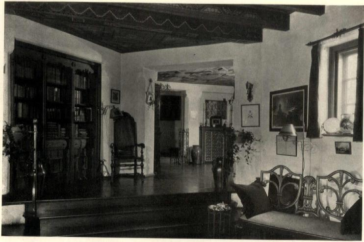
The upper end of the living-room, looking into the reception-room beyond. The walls throughout are sandfloat plaster, left natural for the most part, but painted in several rooms to meet color schemes. The floors are of oak plank secured with wooden dowels
