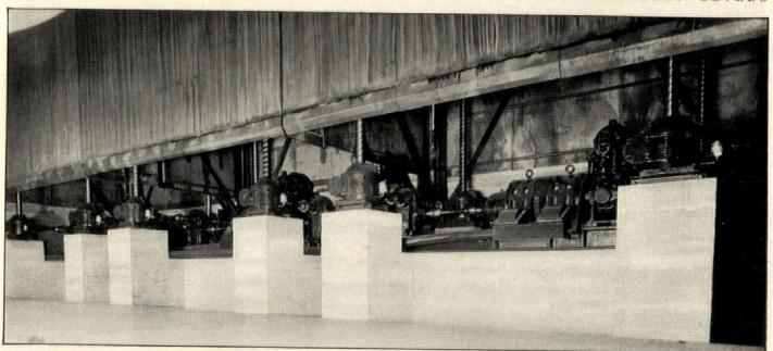
O VIEW OF THE SYNCHRONOUS STAGE-LIFT APPARATUS UNDER THE STAGE
