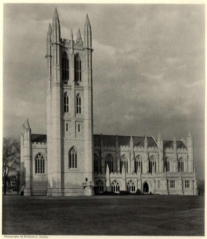
Indiana limestone has been used for the chapel, with a roof of slate. There will be noticed, at the base of the tower, an outdoor pulpit
