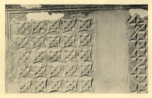
One of the favorites in Essex plaster is this adaptation of the guilloche. A tool is swung from left to right, and by working downwards accuracy does not matter greatly, for each stroke corrects the irregularities of the one above it. The last step is to smooth out and true up the stiles
