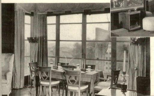
A corner window in a bedroom. The sash, of steel or aluminum, operates separately, to give maximum ventilation. Below, the modern note is carried out in black structural glass.
