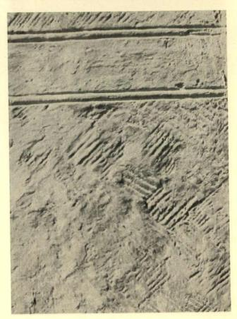
The texture detail to the right is from Ickleton near Saffron Walden; the raw sienna plaster is scored into panels and these in turn marked diagonally in checkered formation. On the opposite page the detail hails from Saffron Walden; here the stile scoring forms curved panel mouldings around the crescent surfacing
