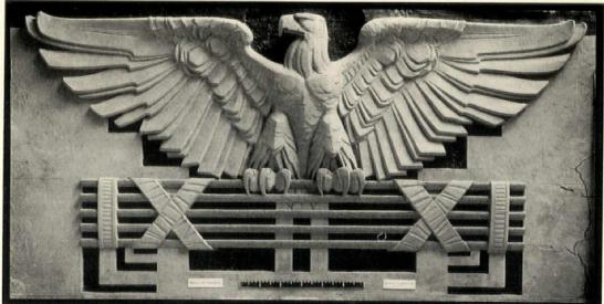
Above, plaster models by René Chambellan of the sound amplification outlet above the proscenium. These were carried out in plaster
