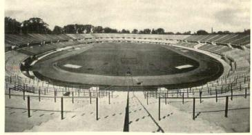
The new Vienna Stadium, to seat sixty thousand people in a great open oval. The architect, Otto Ernst Schweizer, utilized the fine old trees of an existing park. Reinforced concrete is the material used. The upper tier of seats is reached by staircases, the lower tier by tunnels leading from the glass-enclosed ground floor
