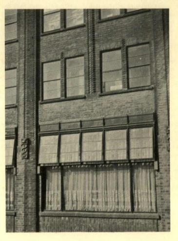
accompanying sketch (left) indicates the skilful manner in which this pier is laid. The intermediate piers and mullions carry the vertical enrichment across the façade, and prevent its being stranded on the widely spaced large piers. The color of the brick varies from pinkish red to yellow ochre. Below, a detail of the intermediate piers
