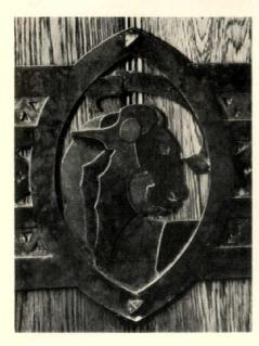
One of the hinges for the main entrance door. There were eight of these, the symbol in the vesica form changing. Two of the variations are pictured at left and right, with the four plates of the eagle superimposed below.
