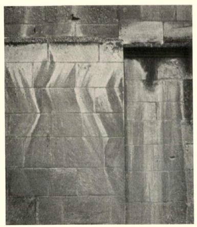
Perhaps one of the least expensive and least appreciated means of stone ornamentation is that of tooling. This detail, from the left nave of Nevers Cathedral, shows how the direction of tooling varies the weathering stains
