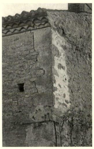
Above—near Bellac (which lies between Limoges and Montmorillon) it is not uncommon to see such cornices as this, of red tile alternating with brick stretcher courses. The interstices of tile ends are filled with gray mortar of the same shade as that which covers the rubble stonework. Gable ends are close-cropped
