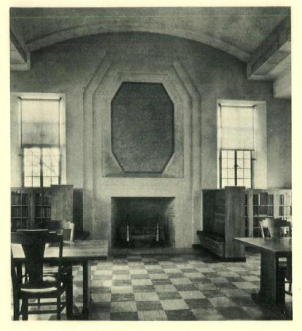
Reading-room at night. Built-in lighting in the ceiling is an innovation proposed by the architects which has proved to be very successful. It eliminates both lights on the tables with their resultant eye strain and clumsy and inefficient chandeliers. Neighbors leave their homes in the evening to come and read in the library on account of the good light
