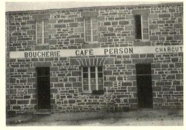
Left—the lintel and bevelled jambs of this little window at St. Jean du Doight are both good design and good masonry. Where roof and wall meet, only cement is used
