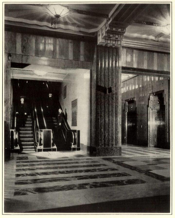
WISH to direct your attention to this photograph because it illustrates an important building trend of today, namely, the use of escalators to supplement elevators. These escalators handle the heavy traffic of lower floors and leave the elevators free to serve upper-floor tenants. Photograph of the new Cities Service Building, of New York City. Sixty Wall Tower. Escalator and elevator installation by Otis Elevator Company.
