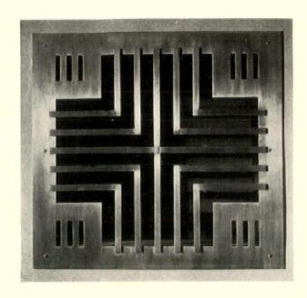
The grilles on this page are fabricated from monel metal in the manner moderne. The one above is composed of sheet material and bars, the one to the right of sheet and strips, while the one below is cast. In addition to not rusting, another advantage of monel metal is that certain parts can be polished brilliantly like nickel, while others can be left a dull gray; practically no upkeep is necessary. Made for the store of T. Eaton & Company, in Toronto, as are those on the opposite page
