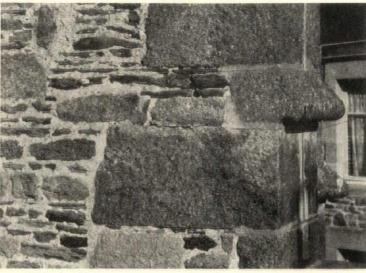
This detail, from a turret on the picturesque ramparts of Mont St. Michel, has coarse, buff mortar, golden-brown granite quoins from 9" to 10" high, and small units of shale varying from slate-colored gray to deep rust
