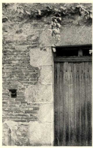
Above—also from Bellac is this detail of a most harmonious and mellow combination of colors and materials: door is weathered brown, granite quoins are in general warm gray, and brick are a soft vermillion. The grape vine has been sprayed with a copper-sulphate solution so that faded emerald green is also present
