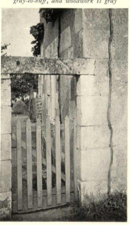
The anatomy of a typical French wall is illustrated by this one at La Charité-sur-Loire, with large quoins and lintel holding in leash a field of small, odd bits. Plaster is then applied so as to finish flush with the quoins
