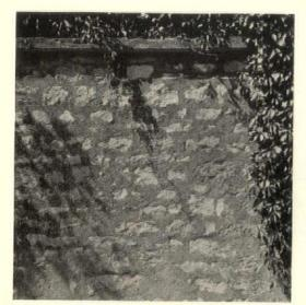
An economic method of using irregular pieces of stone, as well as a means of improving poor jointing, is shown by this warm-toned wall from Vézelay
