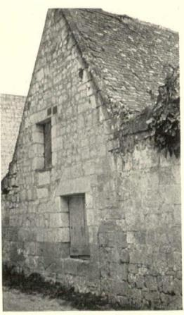
The Cotswolds are rivalled by the Loire in this type of masonry. Note the lack of projecting eaves and the carrying through of horizontal joints
