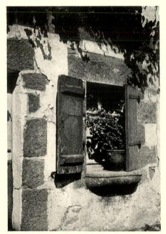
Left—aside from the commendable texture of mortar carried over the stone on this house at Betoulle, south of Bellac, there is a noteworthy cornice composed of a brick soldier course, two rows of curved tile, and one stretcher course. Stone is brown, mortar warm-toned, brick soft red, and shutters brick-red below
