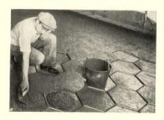
in patented brass strip, nailed to wood underflooring, in tile patterns, 1" thick. Information from National Terrazzo Assn., Portland Cement Assn., or from strip manufacturer, A. C. Horn Company, Long Island City, N. Y.
