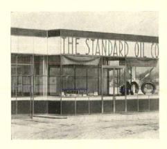
sary. Standard units with verticals and caps, and horizontals, are of stainless steel; panel plates of vitreous enamel in colors. The E. F. Hauserman Company, Cleveland, Ohio.
