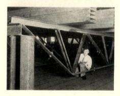
signing the truss so that all members have uniform stress. Diagonal tension members and bottom chord (also in tension) are made from steel straps. Westinghouse Electric & Manufacturing Company, East Pittsburgh, Pa.
