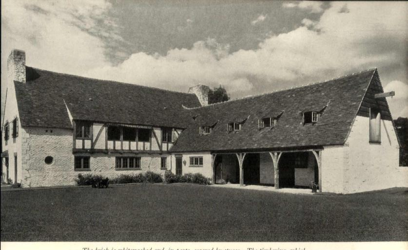
The brick is whitewashed and, in parts, covered by stucco. The timbering, which is structural, is of oak, stained, whitewashed, and wire-brushed after a month or so
