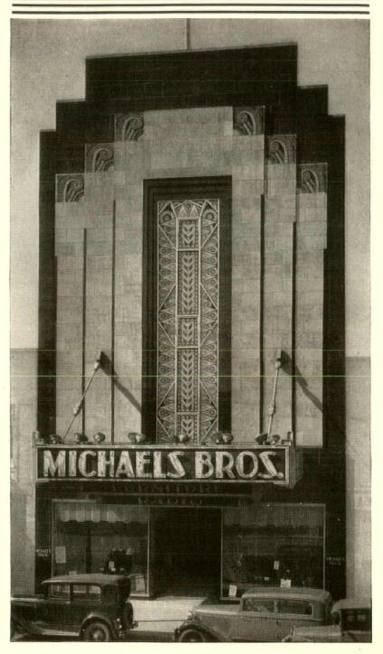
a lustrous glaze. The lighter color is polished aluminum. (The metal is melted and applied at extreme heat directly upon the terra cotta.) The parapet fern decoration is in sparkling polychrome colors...All an unusual bit of modern trade compelling architecture in Terra Cotta.
