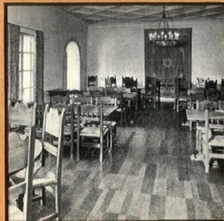
CORK TILE FOR QUIET. Floors of rich brown cork muffle noise in dining-rooms of Scripps College for Women, Claremont, Calif. Armstrong's Cork Tile was used in many other areas, too. Gordon B. Kaufman, architect.
