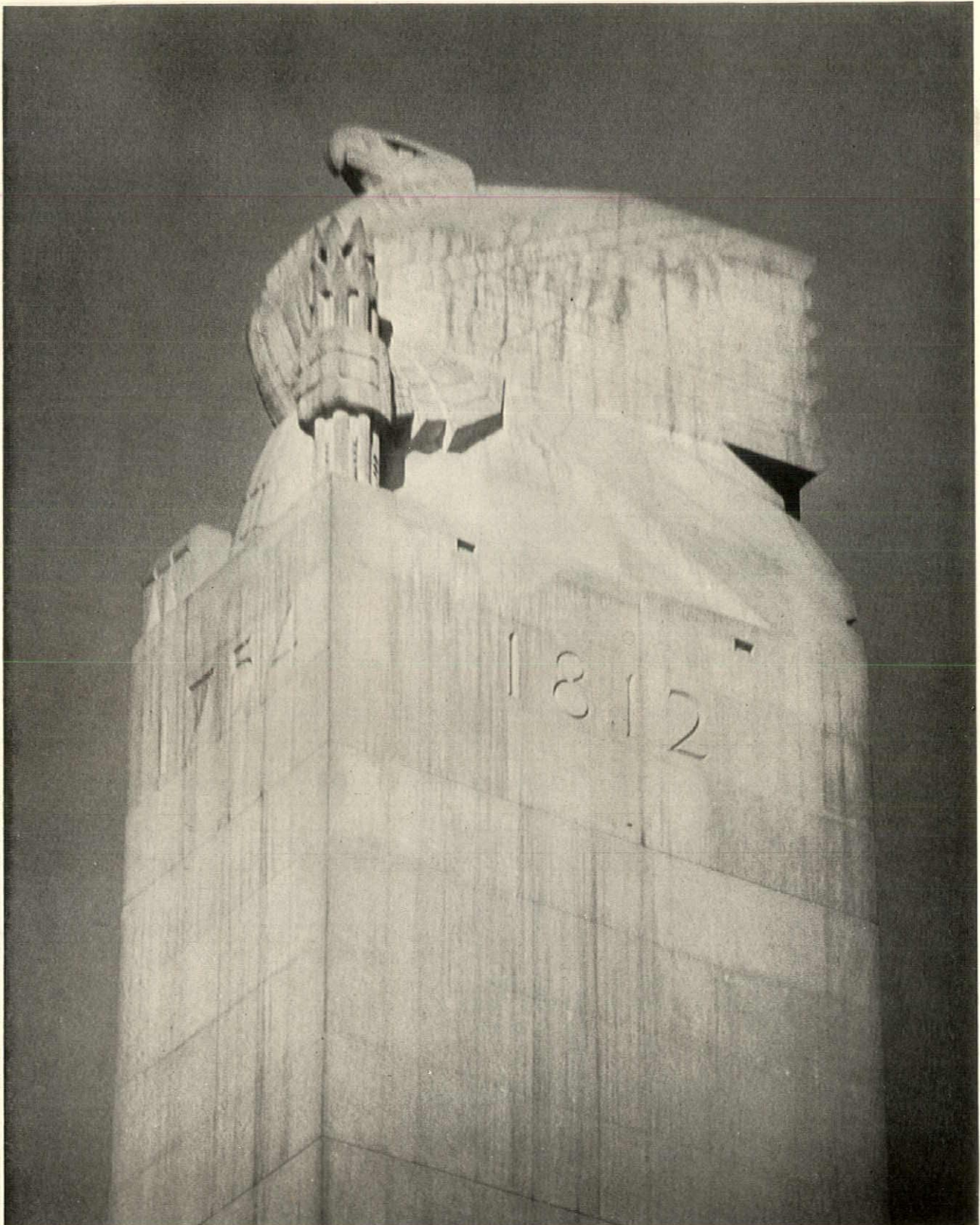
One of the great eagles topping the pylons. Some idea of the scale of this work may be gained from the photograph over-leaf. The pylons are 147 feet high and 16 by 20 feet at the base. For this bridge and the Veterans' Memorial Bridge, Rochester, N. Y., William Gehron, of Gehron & Ross, architects, received the Architectural League's Silver Medal in Architecture for 1932
