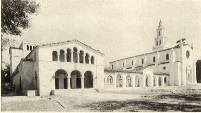
Rollins College, Winter Park, Fla., has just dedicated the Annie Russell Theatre, shown in the foreground (Kiehnel & Elliott, architects), and the Knowles Memorial Chapel beyond, of which Cram & Ferguson are the architects
