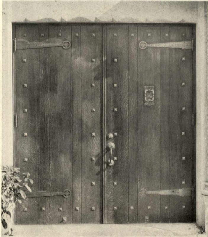
Engineering Department, Southern California Telephone Company
