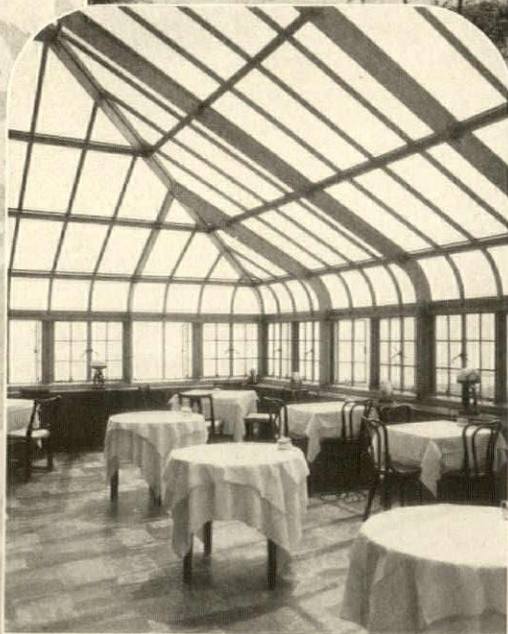
Solar V-Bar Construction on roof of The Kingsley Arms Hotel, Asbury Park, New Jersey
