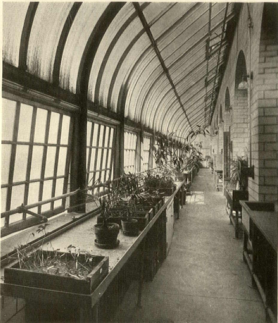
Special design leanto, Central High School, Number 173, Washington, D. C., Wm. B. Ittner of St. Louis, architect.
