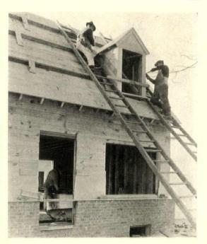
prefabricated, erected by derrick and bolted on. Covering mouldings only to be applied separately.
