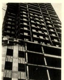
Limestone following the cast alumi-num spandrels up the steel frame. Rockefeller Centre, New York City
