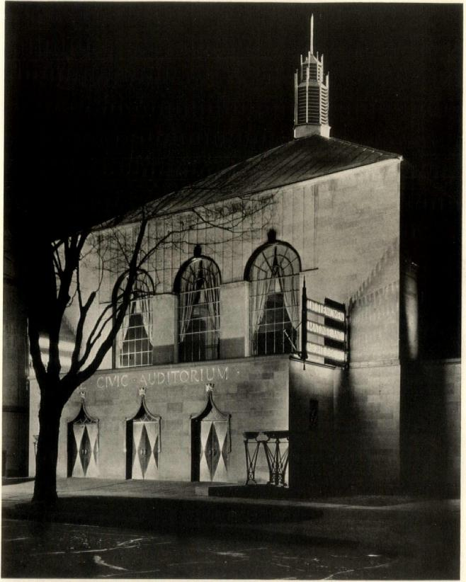
The exterior is in limestone, approaching tan in color; the windows, steel painted with aluminum paint; the doors, stainless steel; roof, copper; flêche, chromium plated. The lettering over the entrance doors is pierced through the limestone, and lighted from behind glass
