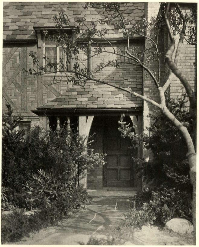
An entrance detail of one variation on the typical plan. The half-timber work with its brick nogging is, of course, genuine
