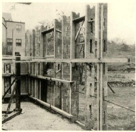
The precast studs are shown in place, a window buck held between two of them by wire under torsion. Note the horizontal rod for reinforcement and the outside form below the window buck
