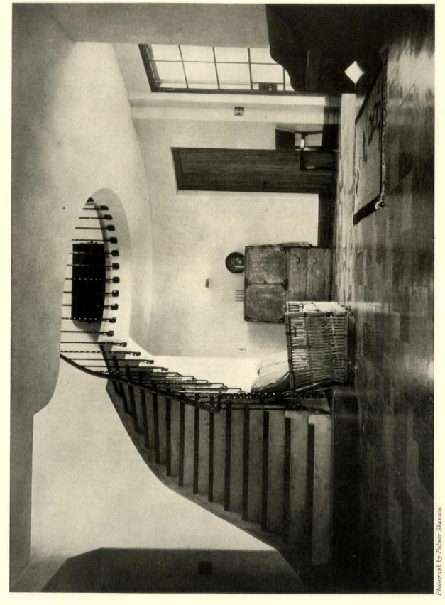
The stair hall. Steps are poured concrete of buff color, with composition tread inserts. Flooring is of composition in buffs and browns with occasional squares in sea green. Ivory walls are obtained by integrally coloring the plaster
