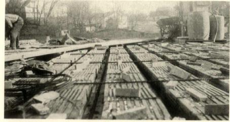
The terra-cotta tile and reinforcing bars in place for the floor slab, ready to pour the concrete. On top of this a composition or tile floor may be laid, or wood flooring on loose sleepers
