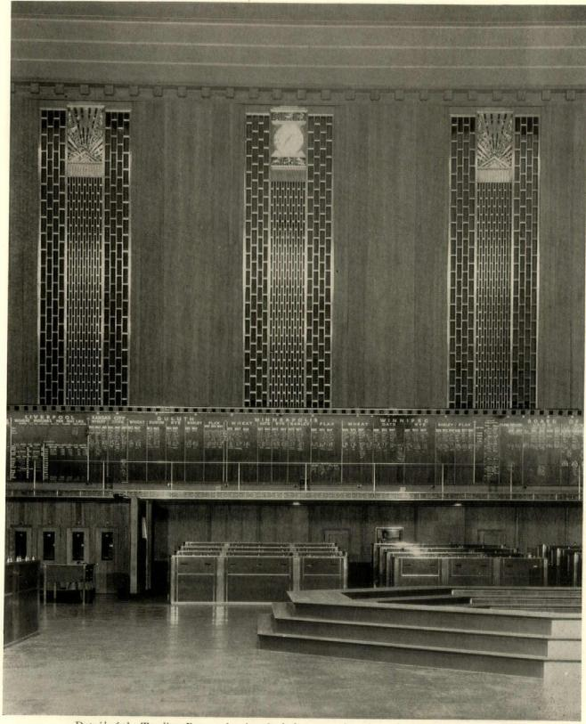
Detail of the Trading Room, showing the balcony overhanging telephone booths and telephone desks, with the quotation board immediately above it. In addition to the soundabsorbing ceiling similar material has been used back of the metal grilles. The room is 111 by 167 feet, 57 feet in height
