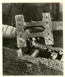
Here is the unit shape, easily grasped by the hand and making a complete eight-inch wall without through mortar joints
