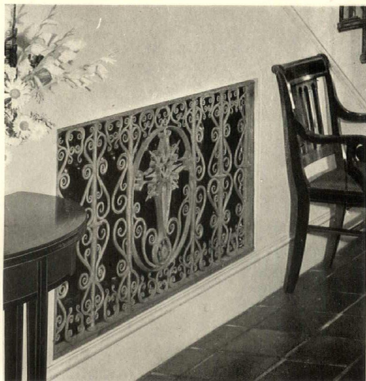
Metal grille as screen under stairs. Delano & Aldrich
