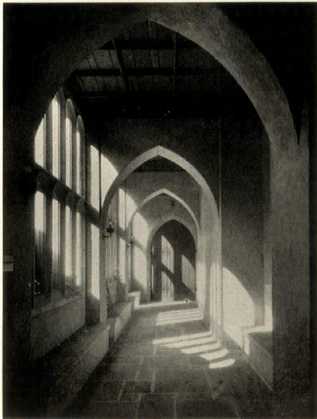
In the North Walk of the Cloister
