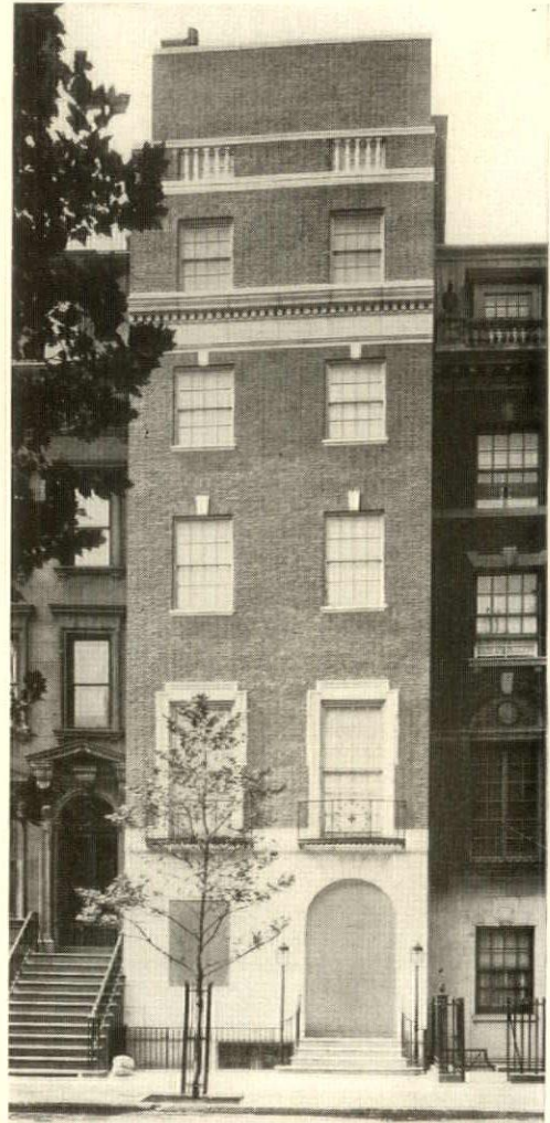
Provision for telephone convenience was built into this well-planned New York residence. EDWARD S. HEWITT, Architect; ROBERT JOHNSON, JR., Builder. The diagram shows the arrangement of the telephones connected to a dial intercommunicating system, with 2 trunk lines and 9 stations, each one equipped to pick up or initiate central office or interior calls.
