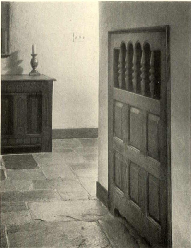
One of two facing convector panels in a hallway
