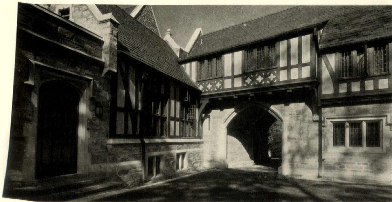
Inside the service court, with the archway entrance in middle
