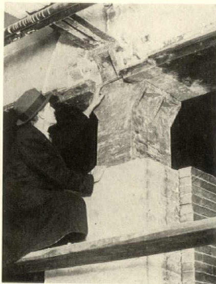
Earl H. Reed, Jr., examining the Home Insurance Building in Chicago to determine whether it was built of skeleton construction
