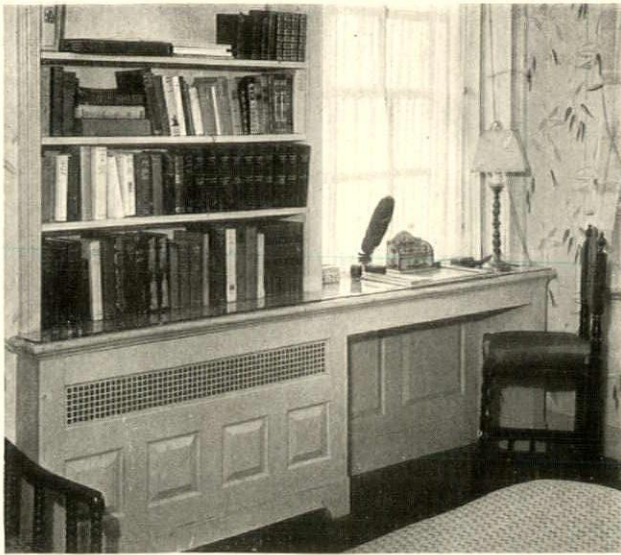
Partly recessed behind woodwork
