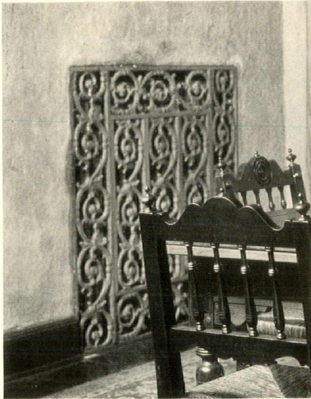
Metal grille to floor, acting as screen only. Moise Goldstein
