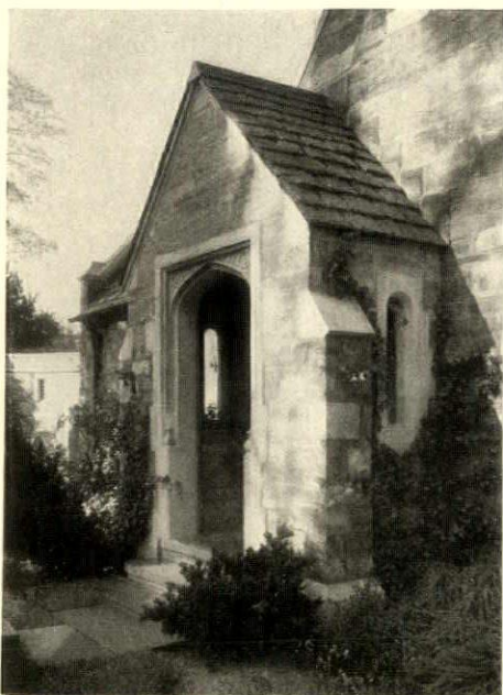
The south entrance to the dormitory, on the upper level
