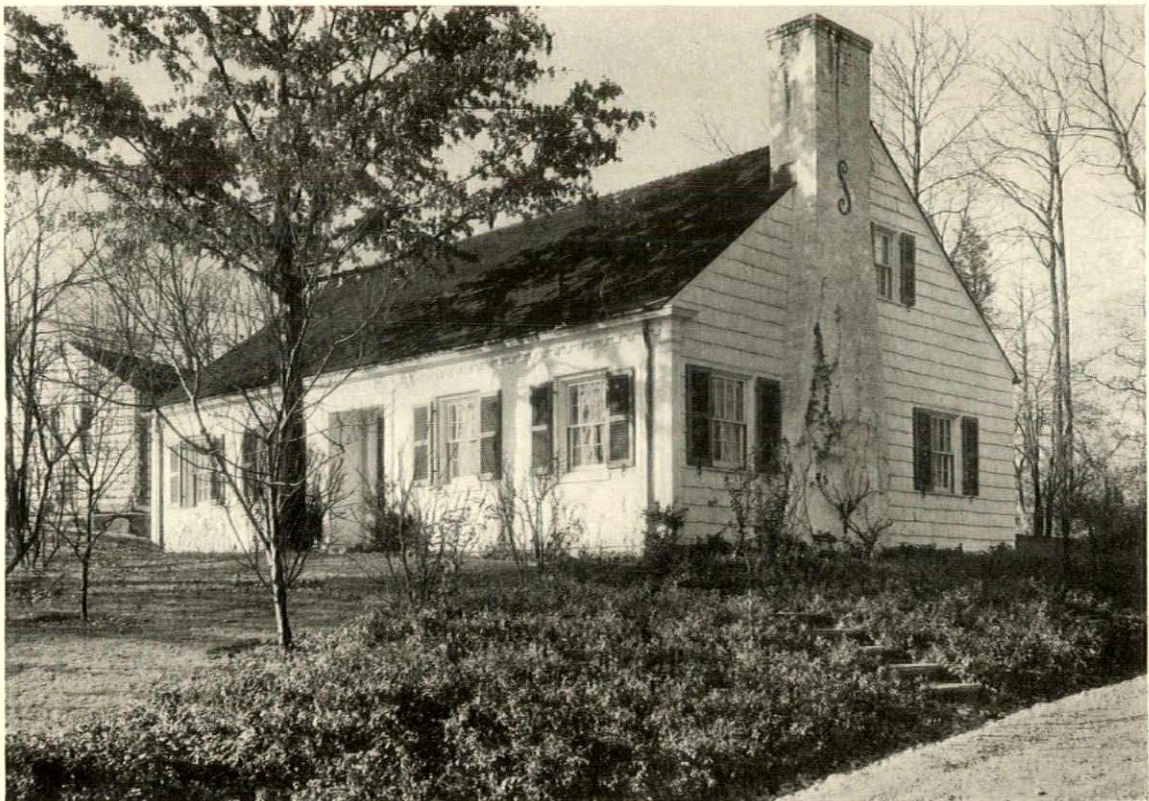
HOUSE OF PAUL D. CRAVATH, LOCUST VALLEY, LONG ISLAND BRADLEY DELEHANTY, ARCHITECT
