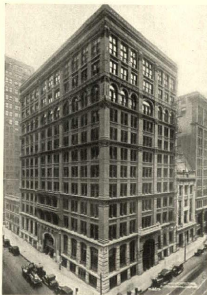
The Home Insurance Building, recently razed, which is designated by an investigating committee as the first high building to utilize the method known as skeleton construction. Designed by William LeBaron Jenney, and built in 1885
