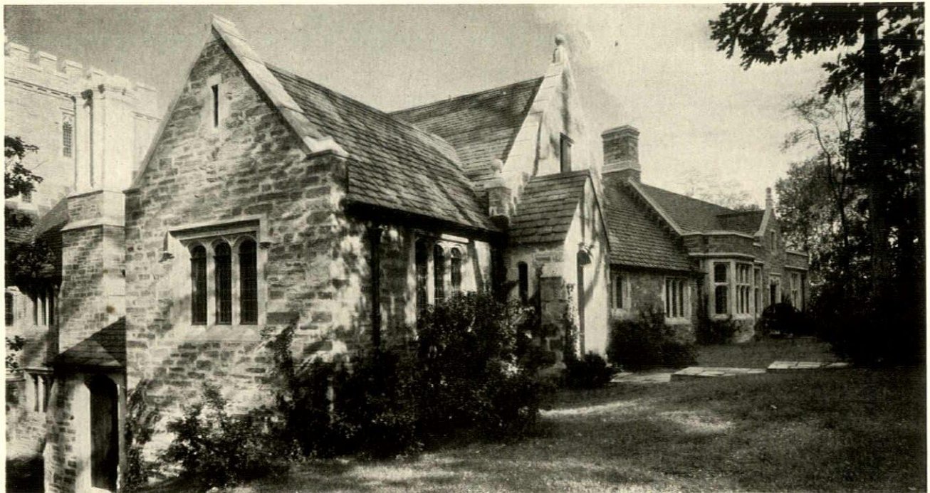
The south wing—dormitory and warden's suite with its entrance on the upper level
