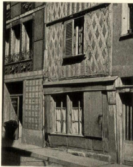
An old house in Chartres, with a particularly lovely texture of brick nogging in the half-timber. Because of the narrow street the photograph had to be taken in two sections
