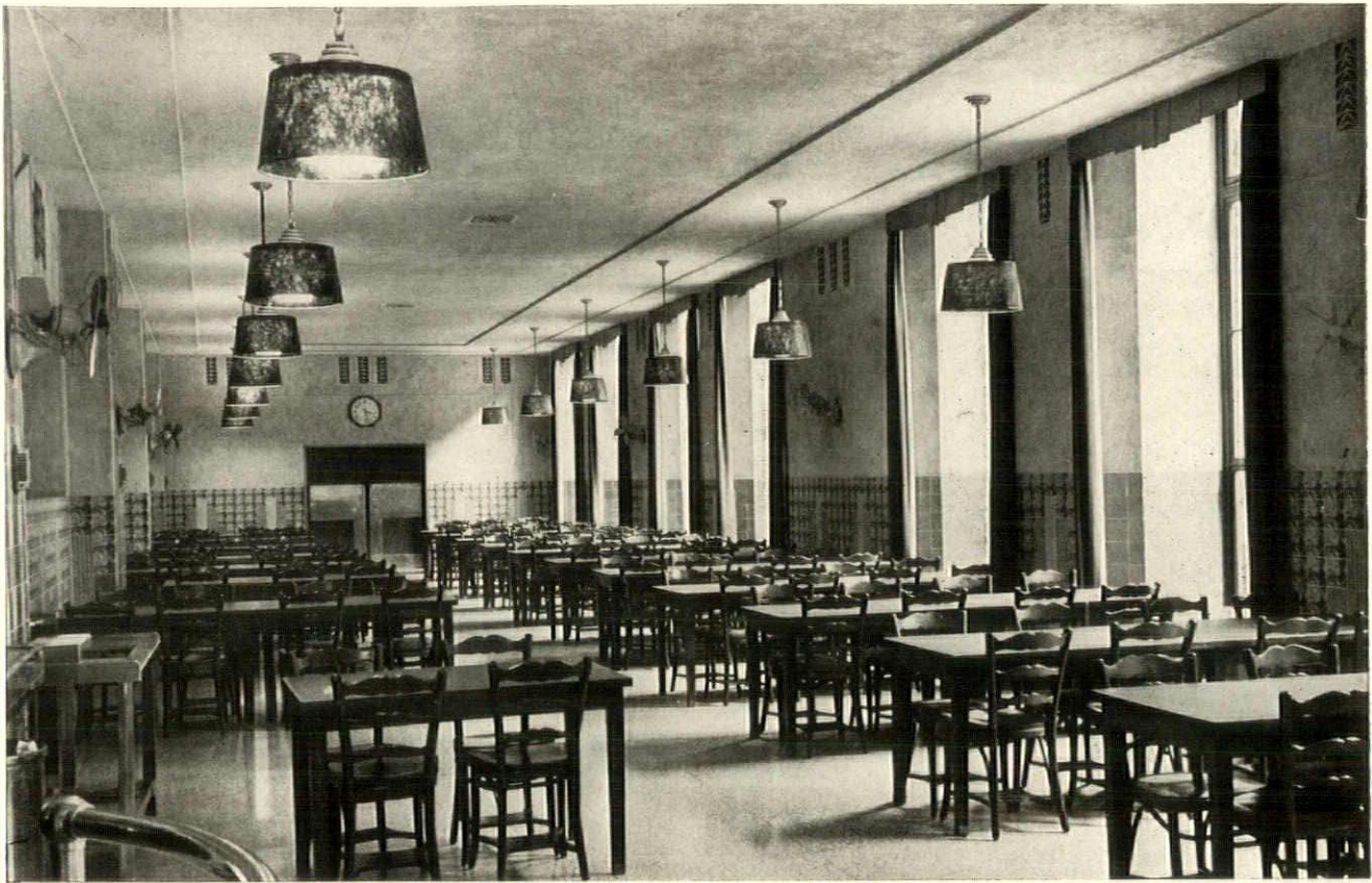
The cafeteria, with its tile wainscot and acoustical plaster above and on the ceiling
