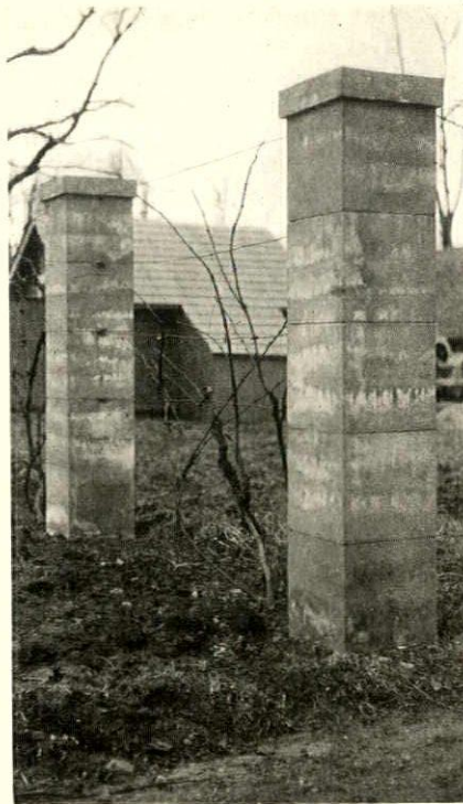
FIG. 9. Below, armored blocks in the fifteen-inch cubes are useful for other purposes, such as fence posts, supporting piers, and the like
