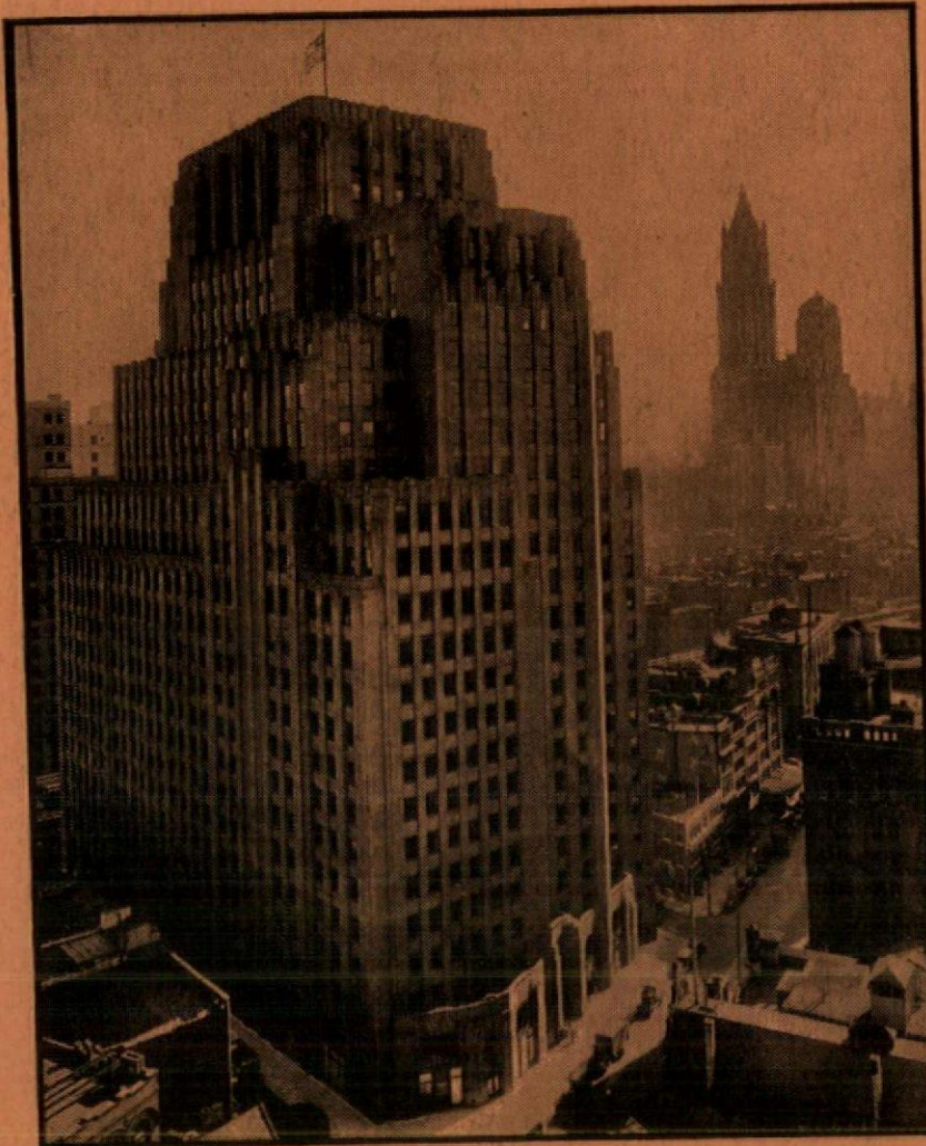
The new Western Union Building in downtown New York at West Broadway, Worth and Hudson Streets. Architects—Voorhees, Gmelin & Walker. General Contractors—Marc Eidlitz & Son, Inc.
