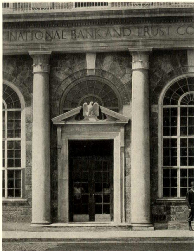
The First National Bank and Trust Company, Mamaroneck, N. Y. Office of John Russell Pope
