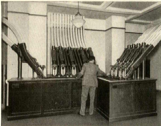
Central Tube Station, State Mutual Life Assurance Co., Worcester, Mass. Parker, Thomas & Rice, Archts. Like in a telephone switchboard, lines reach out to provide communication to all departments.
