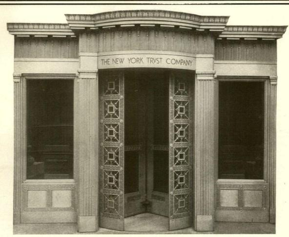
Showing Pocket Curved Door Construction, main entrance N. Y. Trust Co. Cross & Cross, Architects
