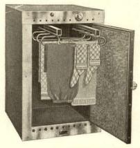
Heat is easily controlled by a 3-heat switch. A ruby pilot light shows whether the current is on or off.
