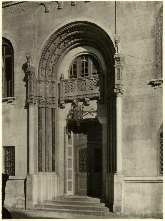
The main entrance of Mr. Baum's West Side Y. M. C. A., where terra-cotta has been used in the splayed reveal with as much recognition of its intrinsic merit as that of the marble colonnettes in the lower part
