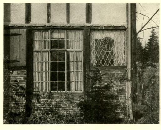
Steel and leaded sash in a timber wall, with decorative lead flashing. W a l t e r Pleuthner
