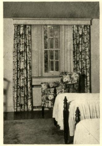
Wood casements, with wood frame screens inside, and boxed head for draperies. Ethel A. Reeve, Inc.
