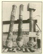
MacARTHUR, Pedestal Type Piles after one of them had supported 50 tons for 10 days without settlement. Note how compressing of concrete has enlarged shaft in pile at left to fill soft spot in soil.
