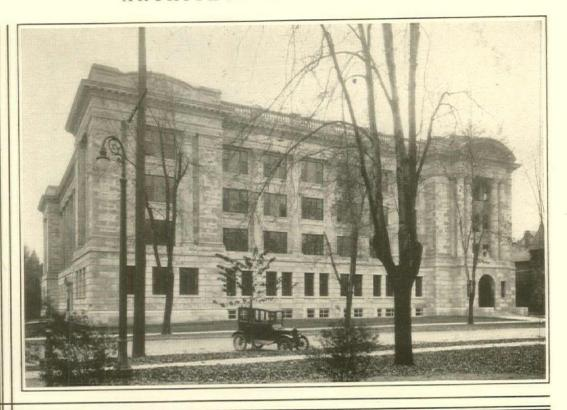
London Life Building, London, Ont., built with Massillon Bar Joist Fireproof Floors and Roof. John M. Moore, Architect. W. H. Yates Construction Co., Contractors.
