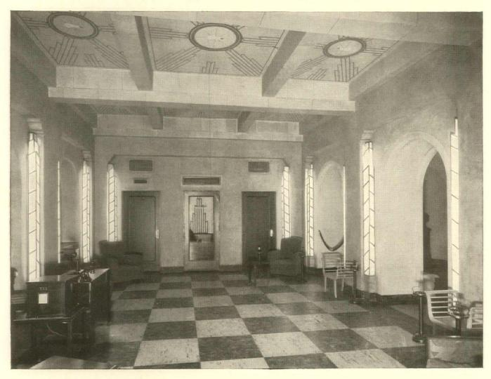
Illumination in this reception room of the Westinghouse Lamp Company's exhibit comes from the Frink illuminated pilasters... The "Solite" glass is evenly illuminated by two vertical rows of Linolite Lamps, particularly well suited for this work because of their continuous filament.
