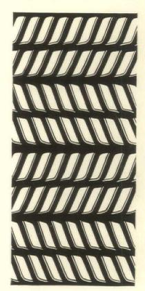
Herringbone mesh with its double rows of steel strands. The unretouched photograph on the opposite page shows the back of a wall plastered on Herringbone Doublemesh. This photograph illustrates how the plaster curls through and around the mesh in opposite directions forming a permanent bond.
