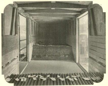
"Central" Conduit is carried into the car one bundle at a time. The larger sizes are placed on bottom and the load is built up until completed. Then it is blocked securely to prevent shifting
