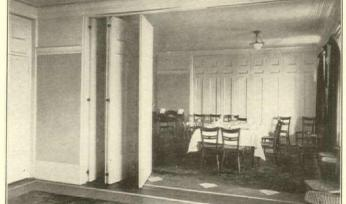
TYPE No. 72 Single hung from center of each alternate door. No track or guide required in floor. For Accordion doors.
