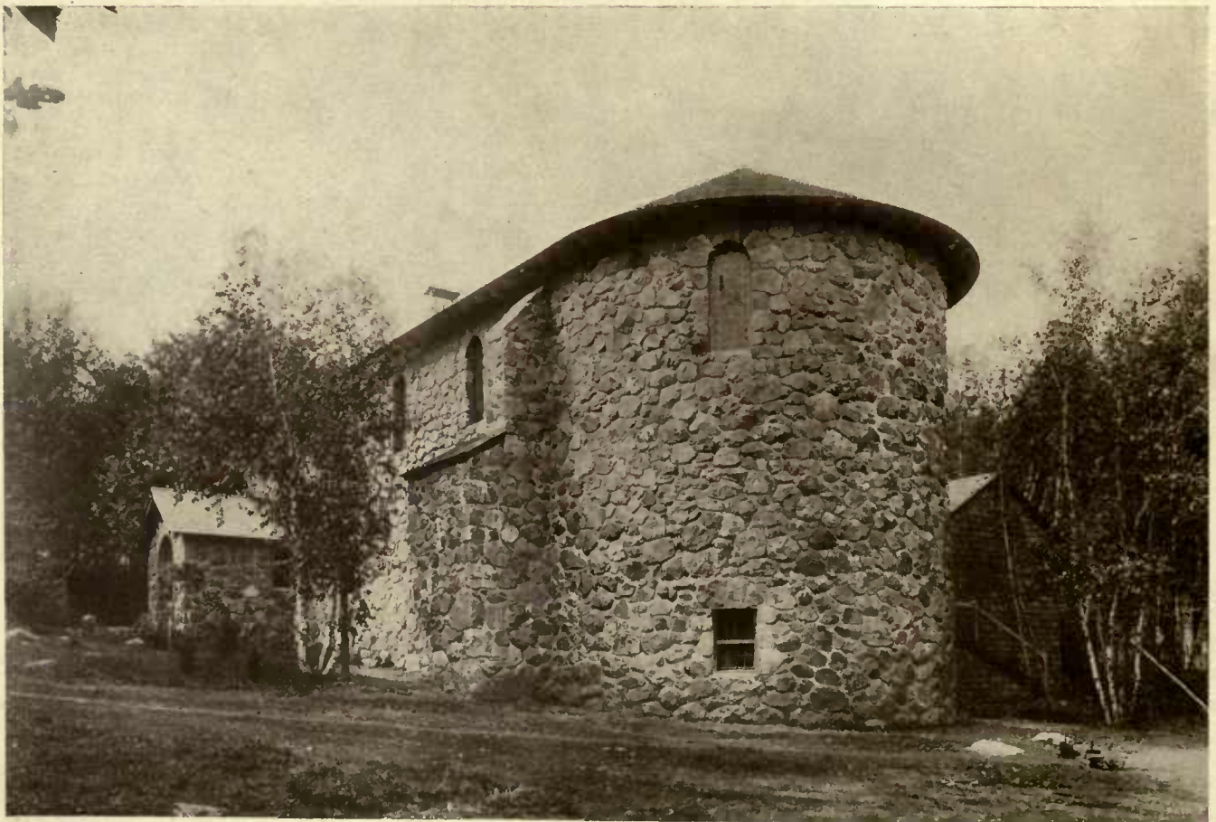
DETAIL OF EXTERIOR.
