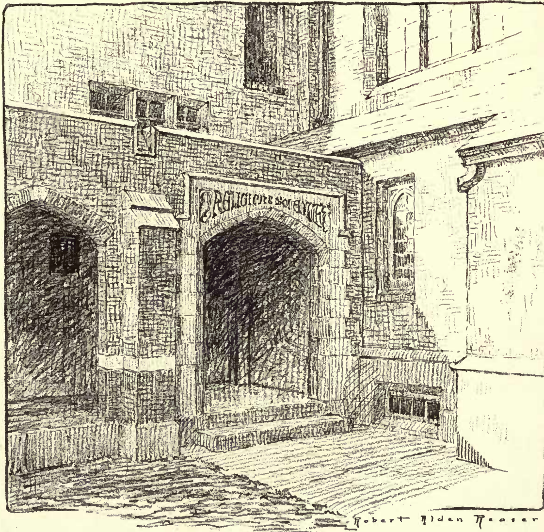
DETAIL OF ENTRANCE TO SCHOOL AND CLOISTER.
