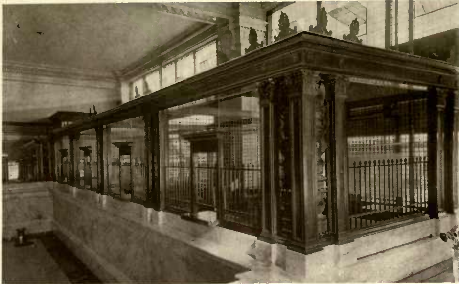
AMBRAC EXTRUDED BRONZE COUNTERSCREEN OF THE BANK OF COMMERCE, SPRINGFIELD, MO. Opel & Torbett, Architects. Fabricated by the Michaels Art Bronze Company, Cincinnati, Ohio, from AMBRAC extruded bronze shapes and mouldings manufactured by The American Brass Company
