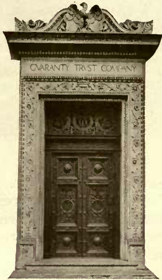
Flanking the entrance of the Guaranty Trust Company's Fifth Avenue offices are exquisite examples of granite carving. York & Sawyer, Architects.
