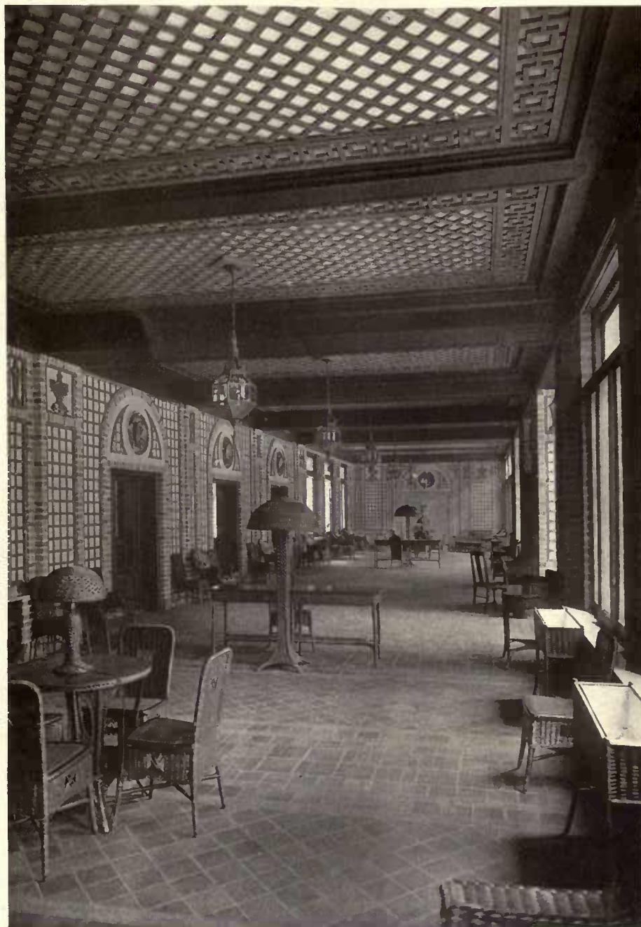
ENTRANCE LOGGIA, FACING 16TH STREET.
