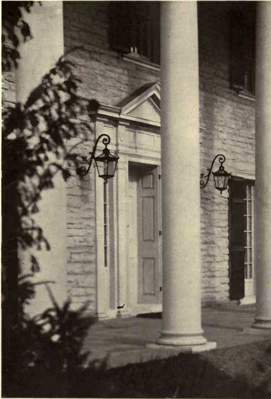
PORTICO AND FRONT DOOR.
