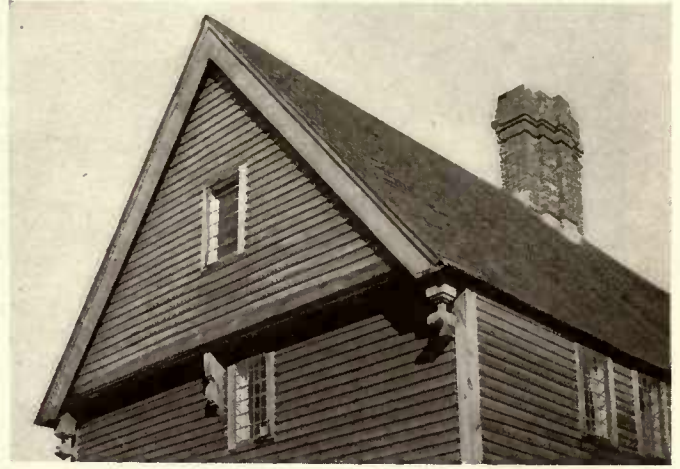
Overhanging gable end with chamfered end girt, bracket and drops; moulded verge board.
