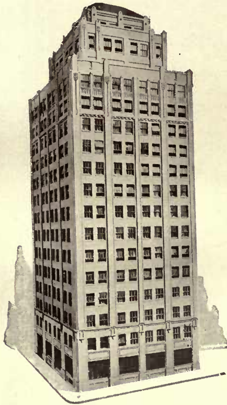
Barrett Specification 20-year Bonded Roof on Hide & Leather Realty Co. building, New York City. Eng. & Gen'l. Cont.: Thompson & Binger, New York; Roofer: New York Roofing Co., New York City.
