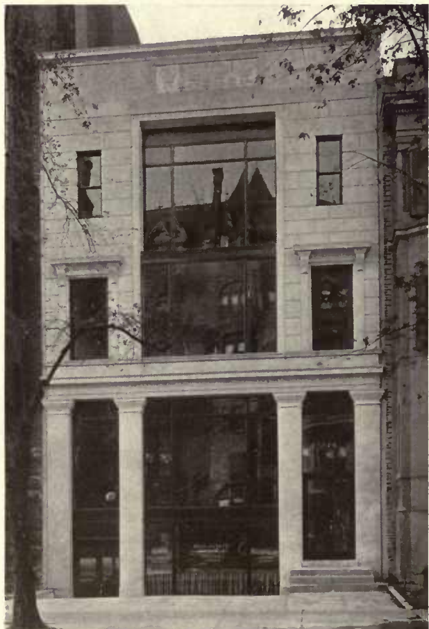
STORE BUILDING, 804 17TH STREET, WASHINGTON, D. C.
