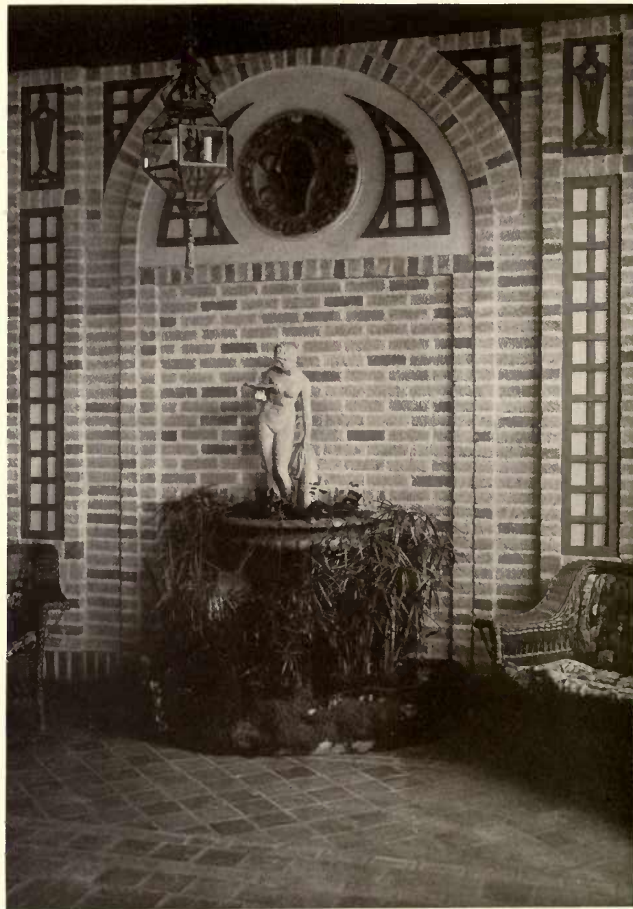
FOUNTAIN IN END OF LOGGIA. (Cast aggregate with medallion of colored terra-cotta.)
