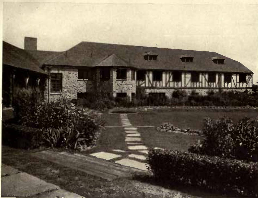
View of garden, showing the end of the dining-room and men's locker-room. A mixture of stone, rustic timbers, and the half timber and stucco, with gray-brown shingle roof.
