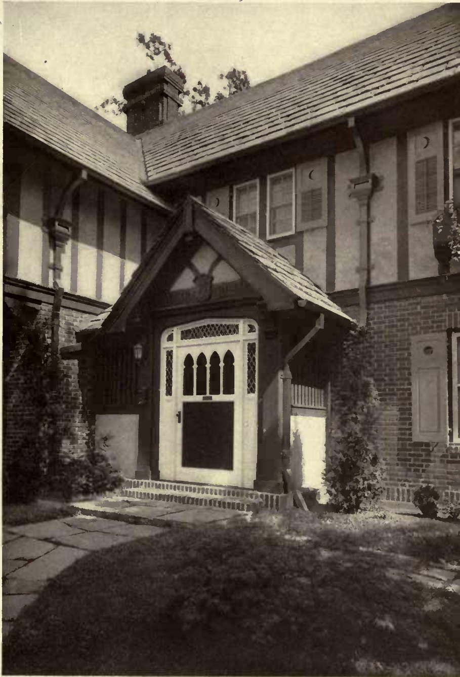
ENTRANCE PORCH, HOUSE, HARRY F. WEBER, MT. VERNON, N. Y.
