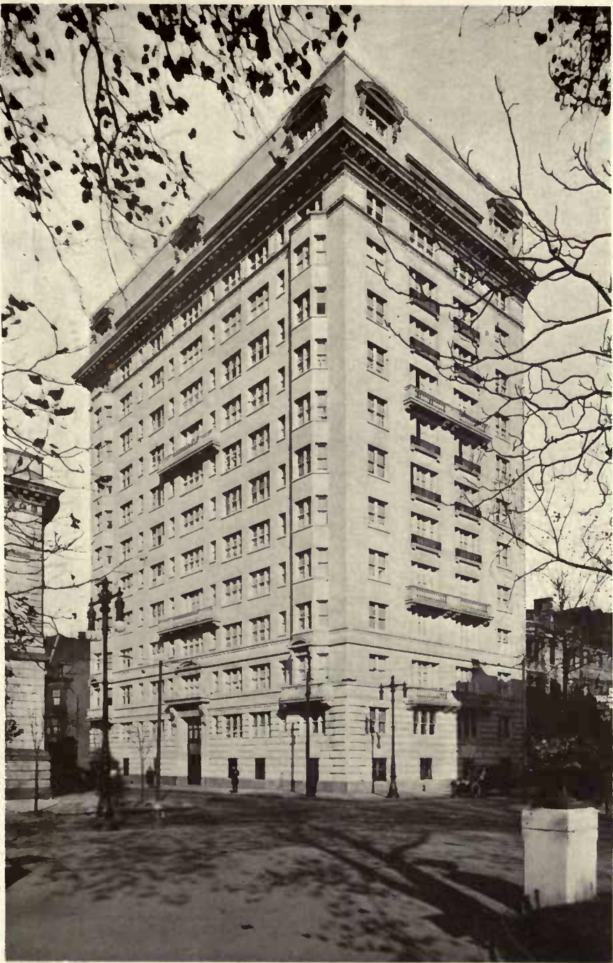
APARTMENT HOUSE, 135 SOUTH 18TH STREET, PHILADELPHIA, PA.
