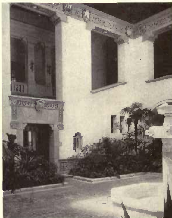
PAN-AMERICAN UNION, WASHINGTON, D. C. Albert Kelsey and Paul Cret, Architects. Gray and polychrome terra-cotta contrasted with white stucco walls.
