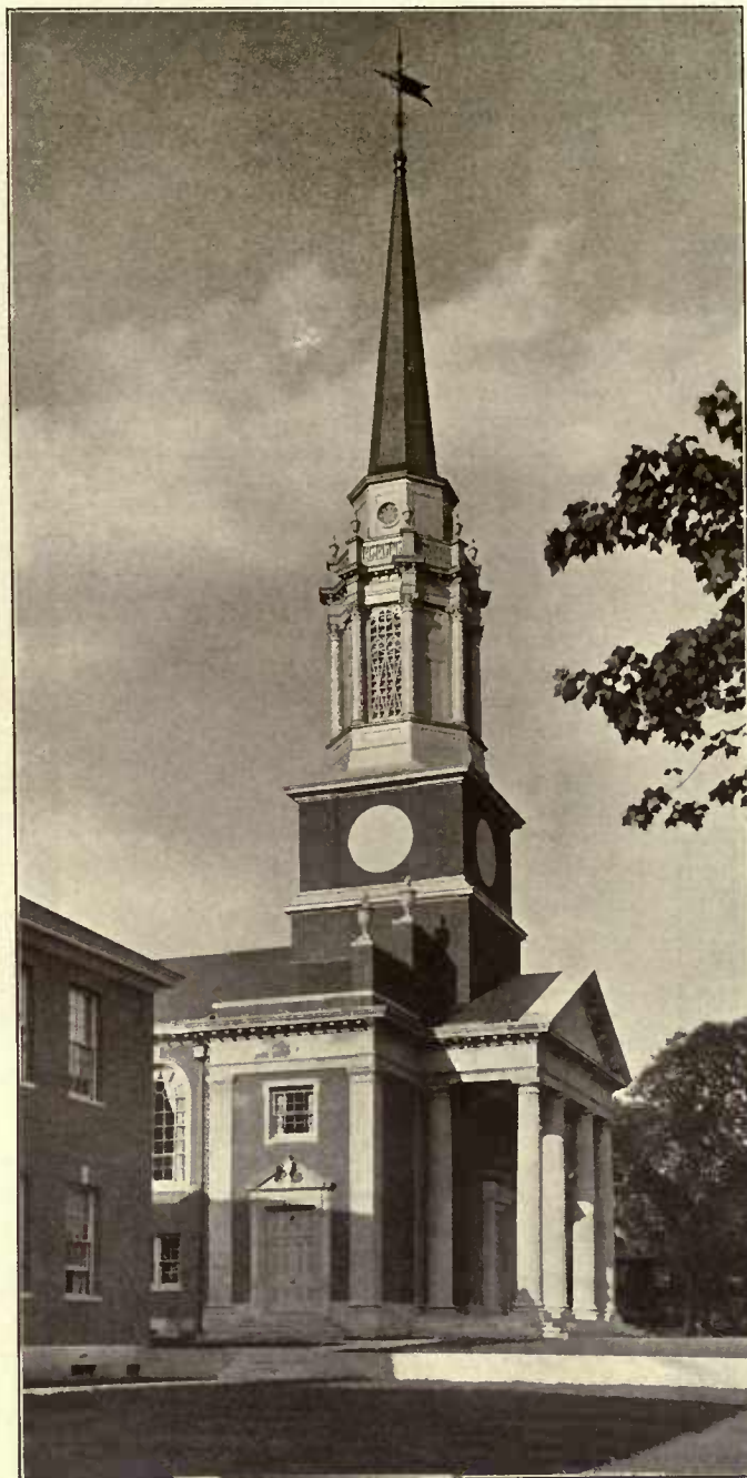
Central Presbyterian Church, Montclair, N. J. Carrère & Hastings, Architects Shreve, Lamb & Blake, Associated
