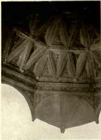
The Artesinado ceiling of the stair-hall, University of Oñate.
