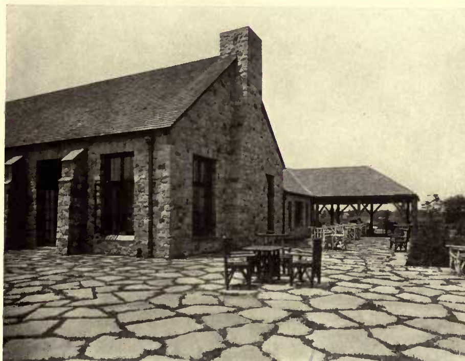
The end of the living-room and entrance porch. The buttresses counteract the thrust of the heavy trusses on the inside of the living-room.
