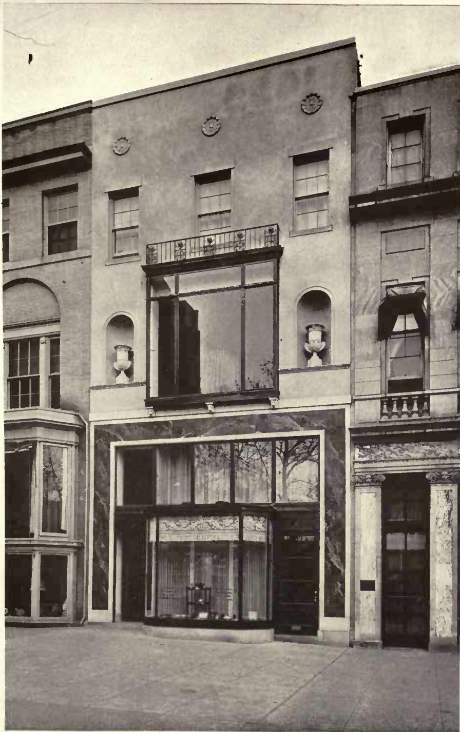
STORE AND APARTMENTS, 1145 CONNECTICUT AVENUE, WASHINGTON, D. C.
