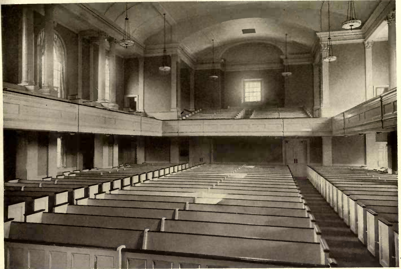
INTERIOR, TOWARD ENTRANCE.
