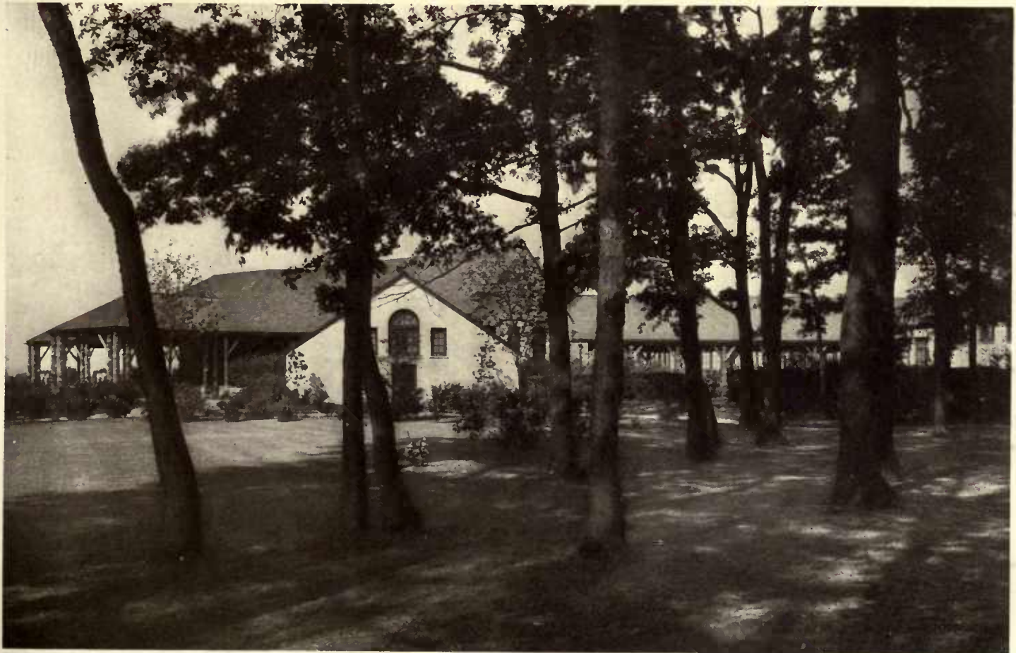
GENERAL EXTERIOR VIEW, WITH PORCH CONSTRUCTED OF RUSTIC TIMBERS. NORWOOD GOLF CLUB, LONG BRANCH, N. J.
