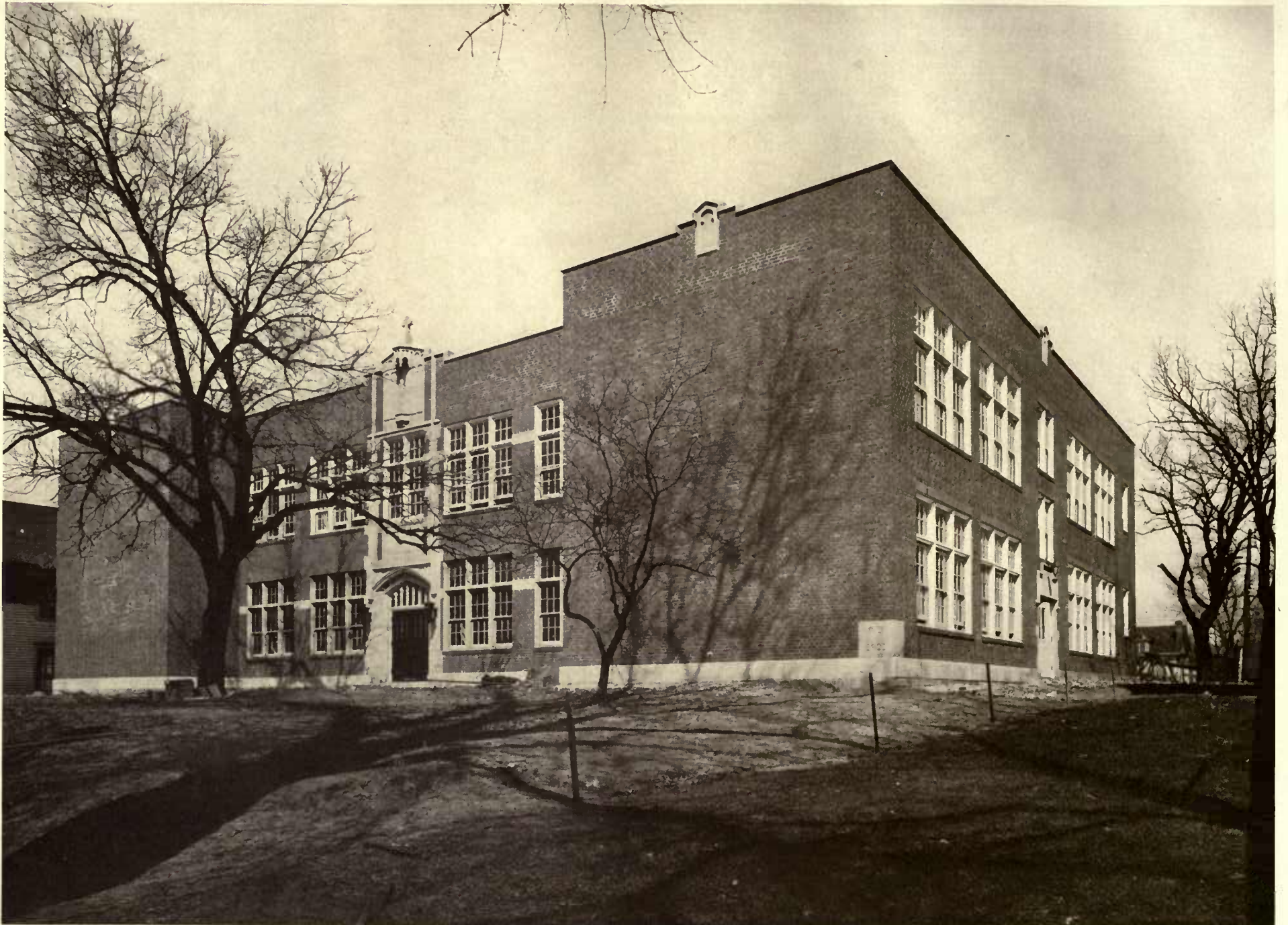
CHURCH AND SCHOOL OF ST. LAWRENCE, R. C., MINNEAPOLIS, MINN.
