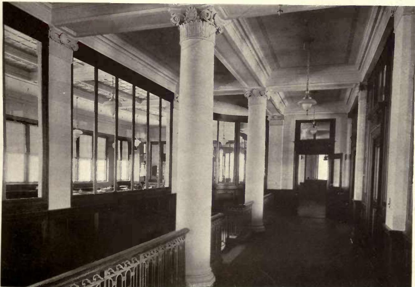
STAIR HALL, SECOND FLOOR.
