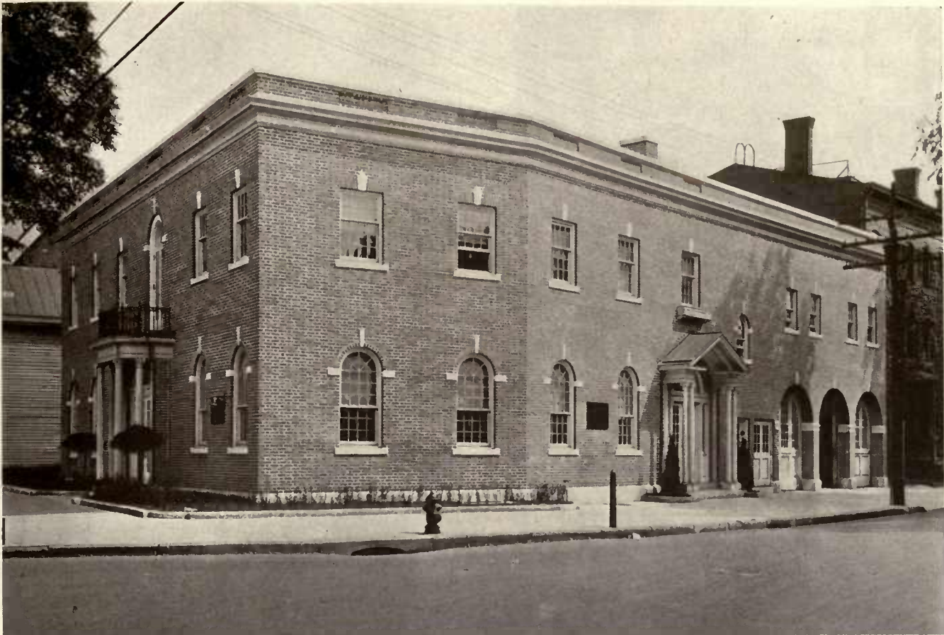
BEECHER & BENNETT BUILDING (UNDERTAKING PARLORS), NEW HAVEN, CONN. Charles Scranton Palmer, Architect.
