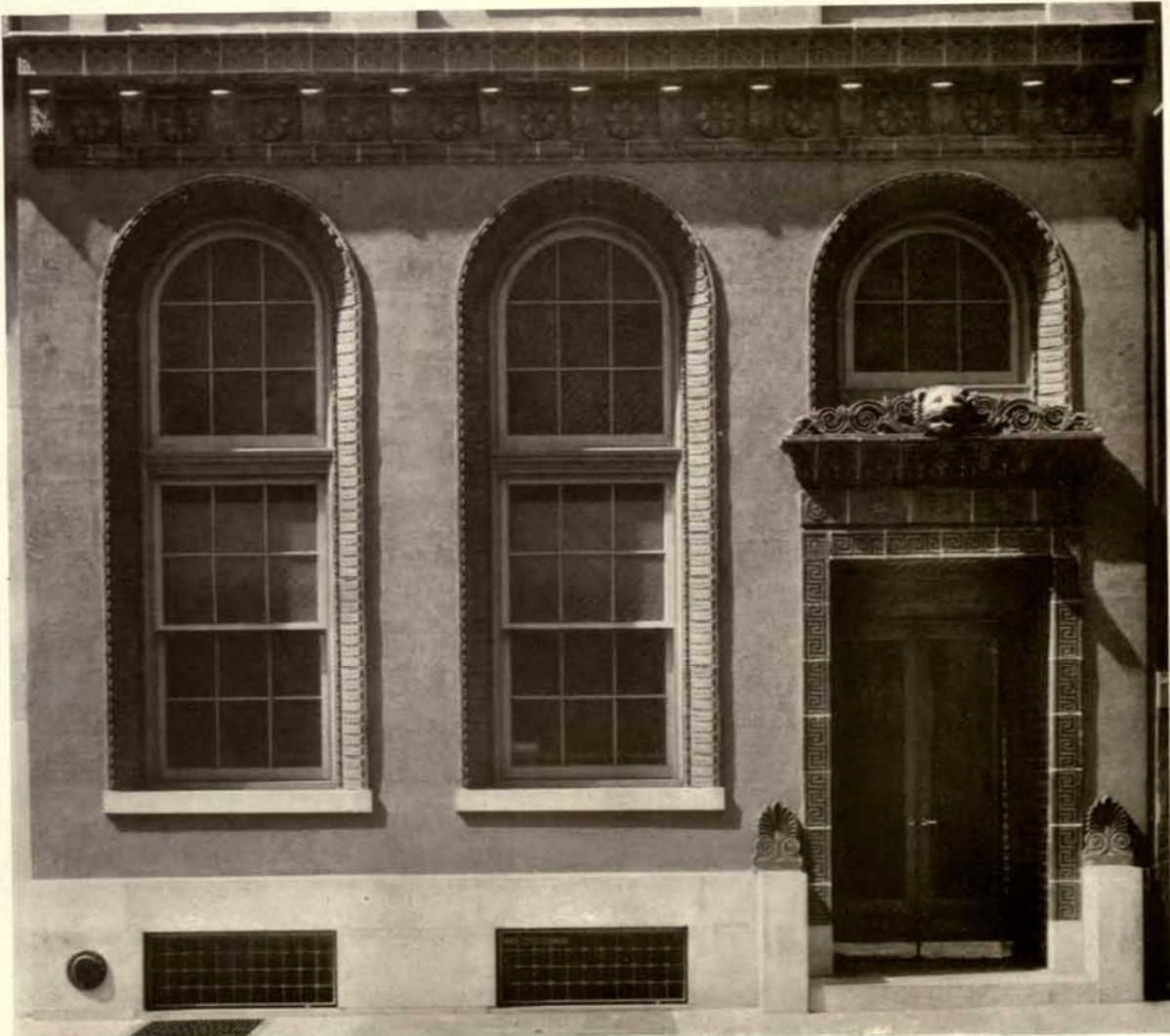
THE BUILDING OF THE AMERICAN ENCAUSTIC TILE CO., 16 EAST 41ST STREET, NEW YORK. Designed by the owners.
