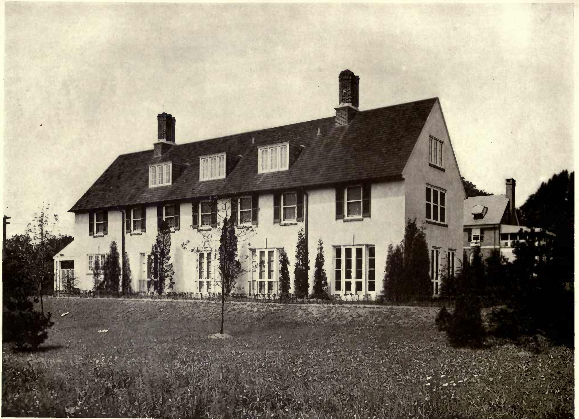
HOUSE, JOHN McMULLIN, OVERBROOK, PA.
