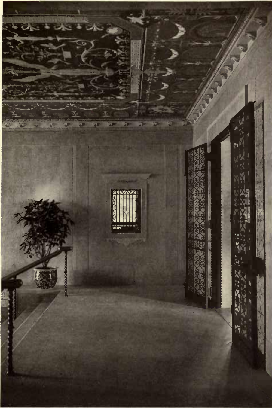
TOP OF STAIRWAY IN ENTRANCE LOBBY.
