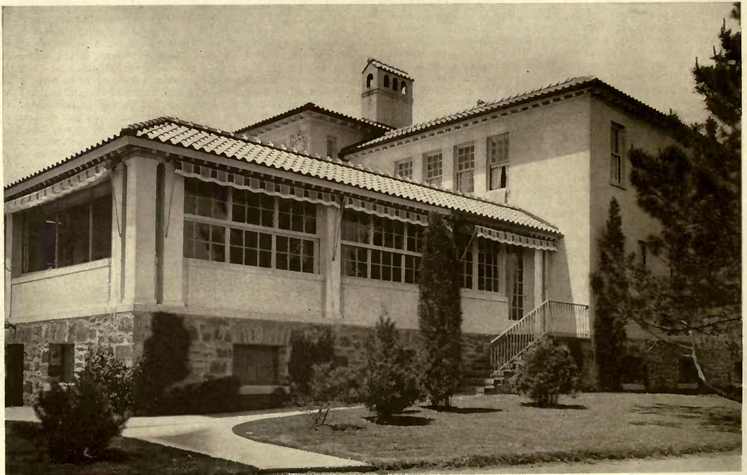
THE LOUNGE PORCH.
