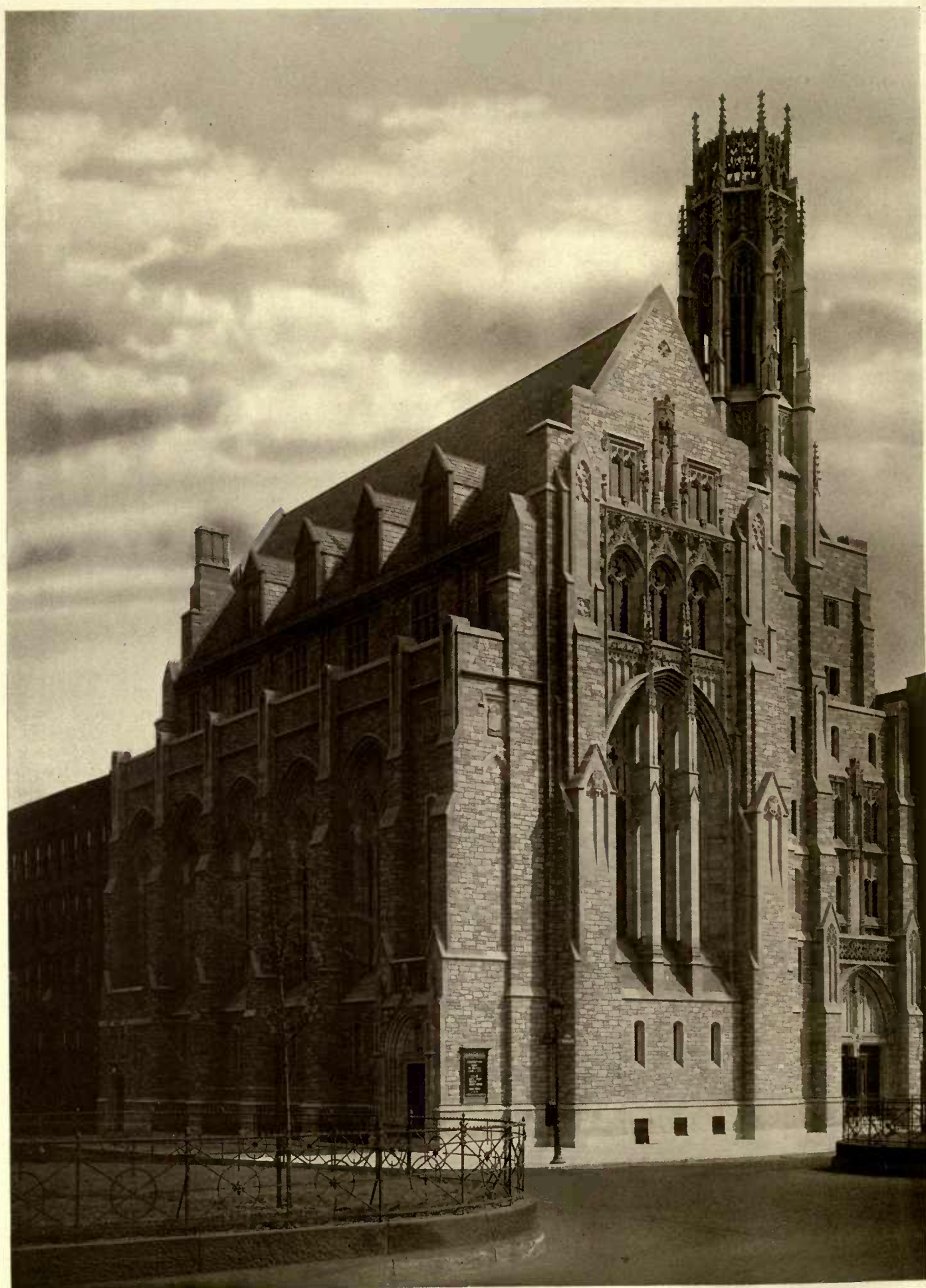
THE PARK AVENUE BAPTIST CHURCH, NEW YORK. Henry C. Pelton, New York; Allen & Collens, Boston, Associate Architects.
