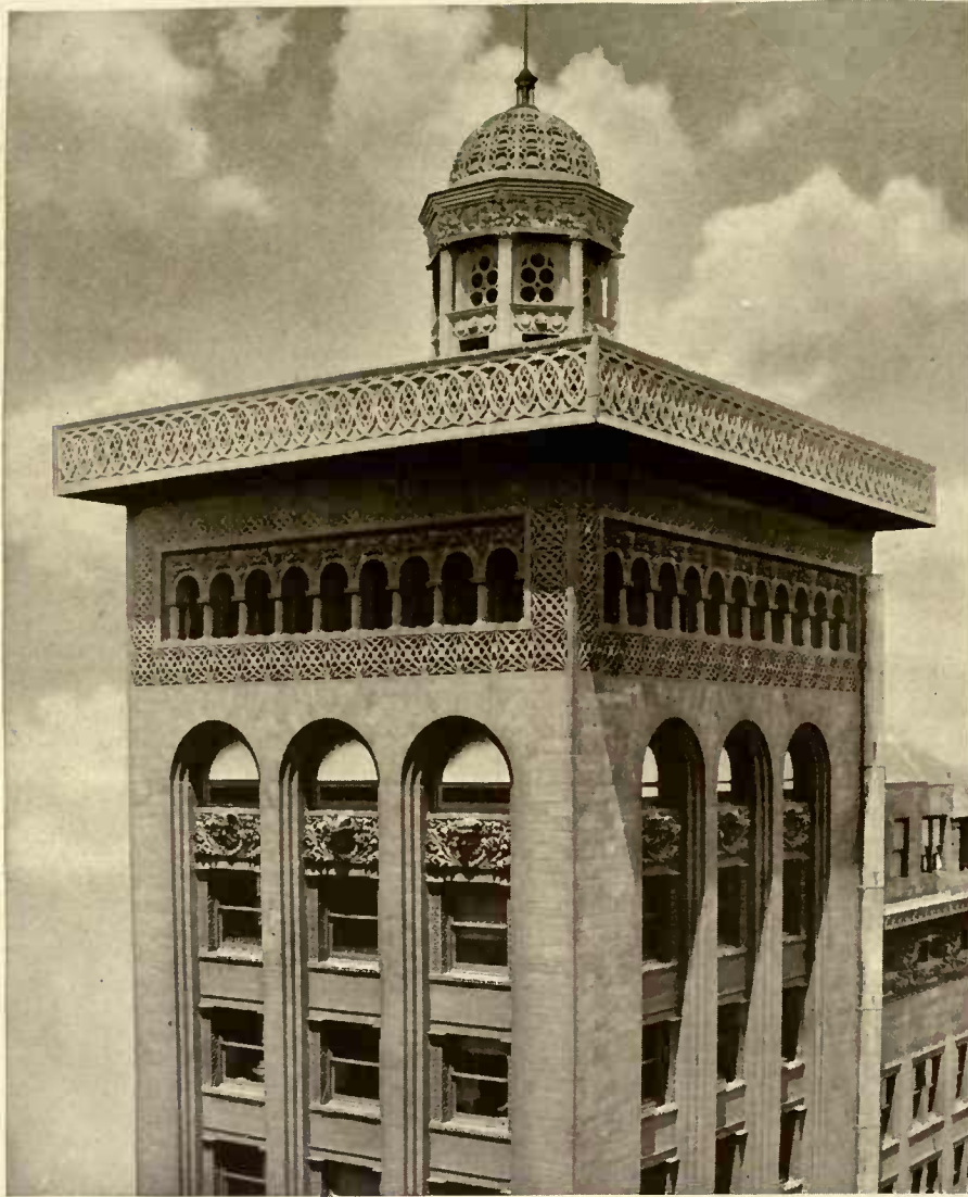
Garrick Theatre (formerly Schiller Theatre) Building, Chicago, Illinois. Adler & Sullivan, Architects. Gray unglazed Terra Cotta throughout. Erected 1891. Photograph taken 1922.
