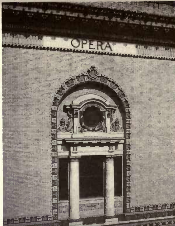
BROOKLYN ACADEMY OF MUSIC. Herts & Tallant, Architects. Window detail of polychrome terra-cotta.
