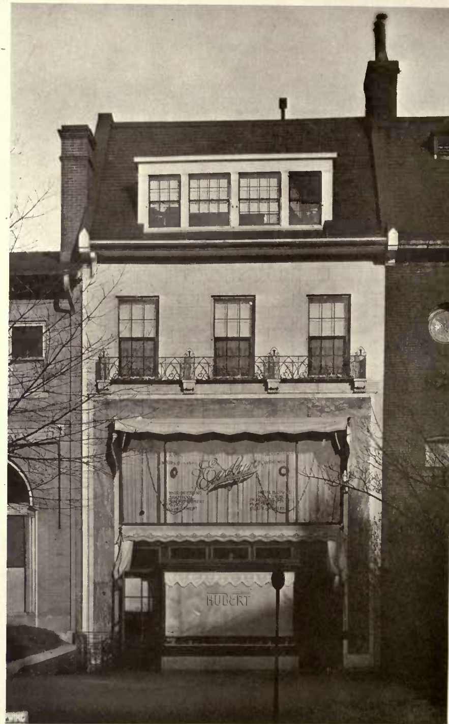
STORE AND APARTMENTS, 1803 CONNECTICUT AVENUE, WASHINGTON, D. C.
