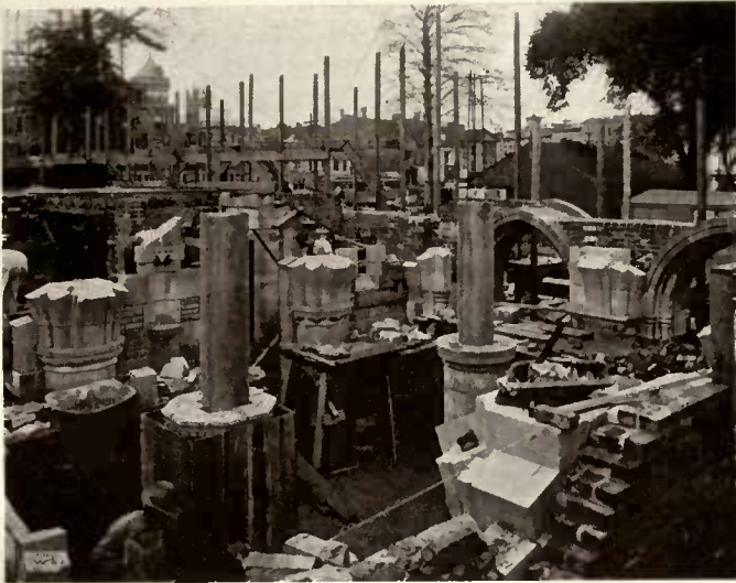
Construction of passage to Calliope Court.
