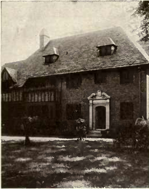
RAPHAEL HUME, ARCHITECT
