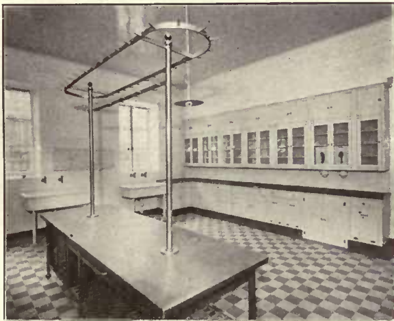
Kitchen showing extensive layout of WHITE HOUSE Units. Note how the wall is furred down and tiled to the top of the Units.
