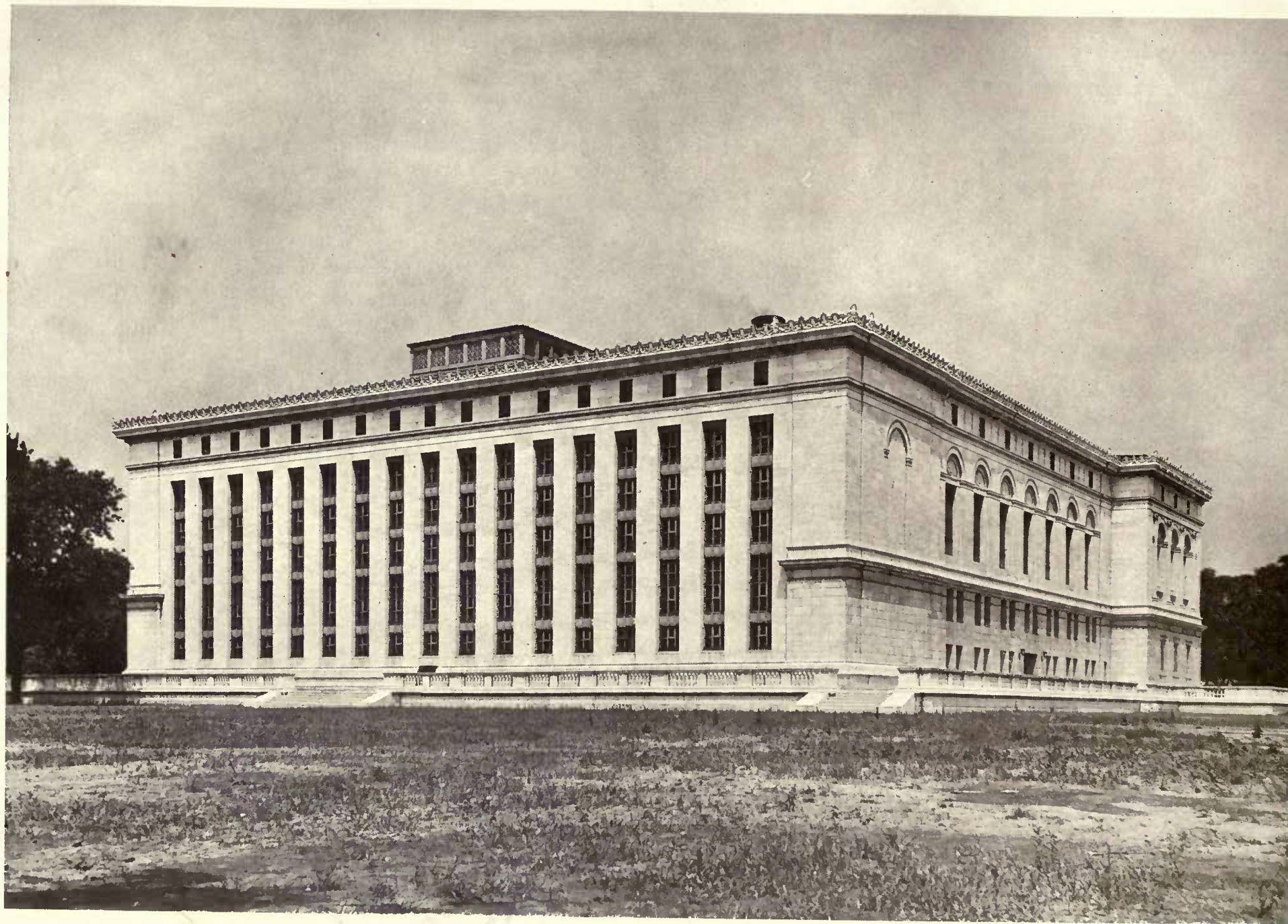
REAR (SHOWING STACKS), THE DETROIT PUBLIC LIBRARY, DETROIT, MICH.
