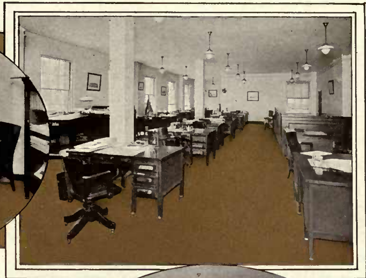
One of the larger offices.
