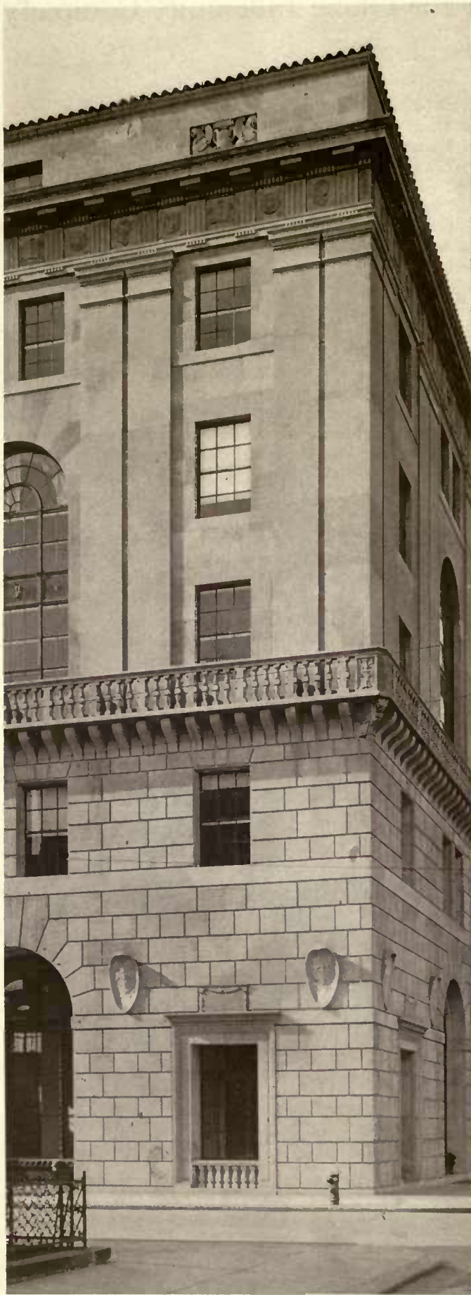
Corner detail, Administration Building, Globe Indemnity Co., Newark, N. J. Frank Goodwillie, Architect. Wesley S. Bessell, Associate.
