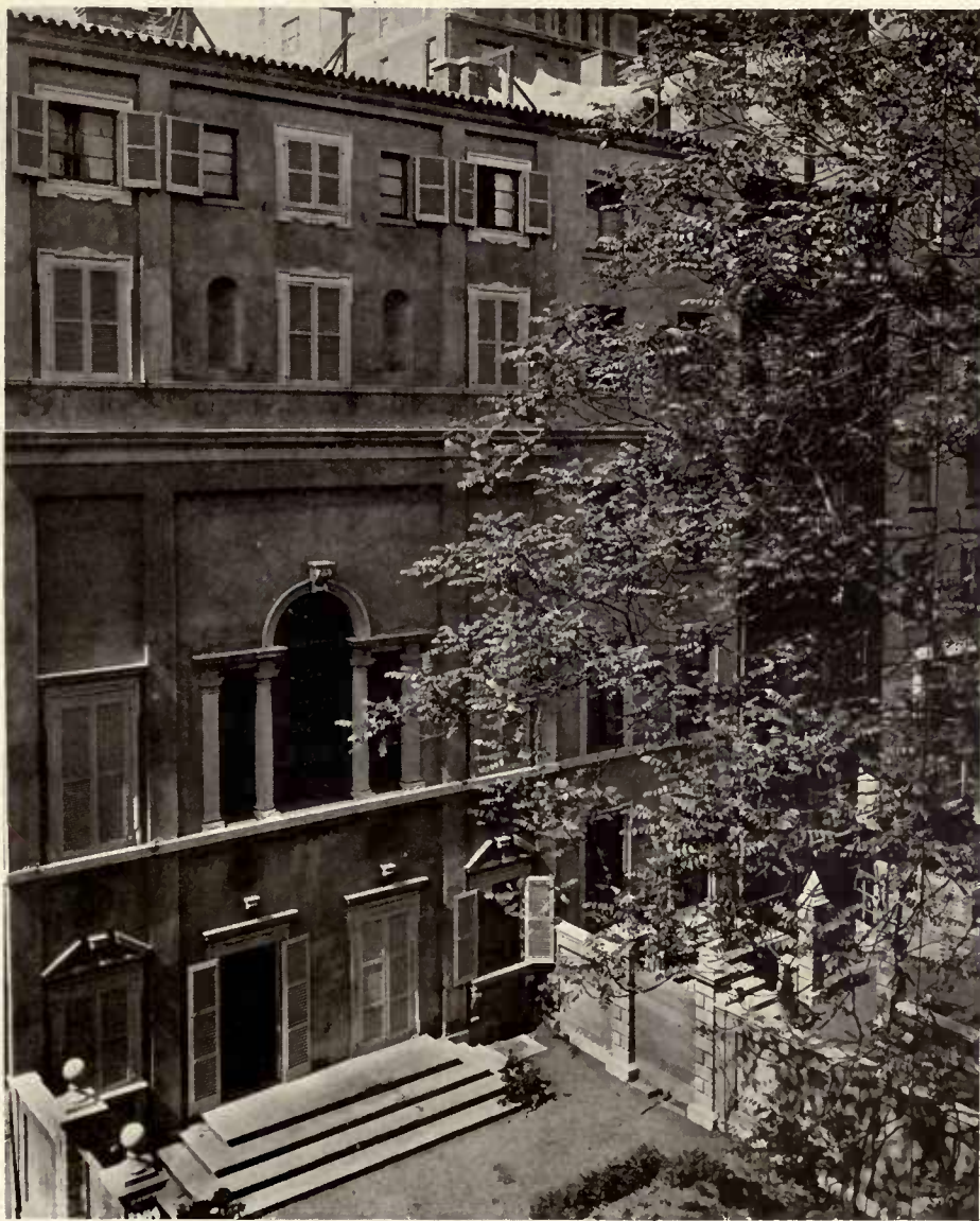
REAR OF HOUSE AND GARDEN.
