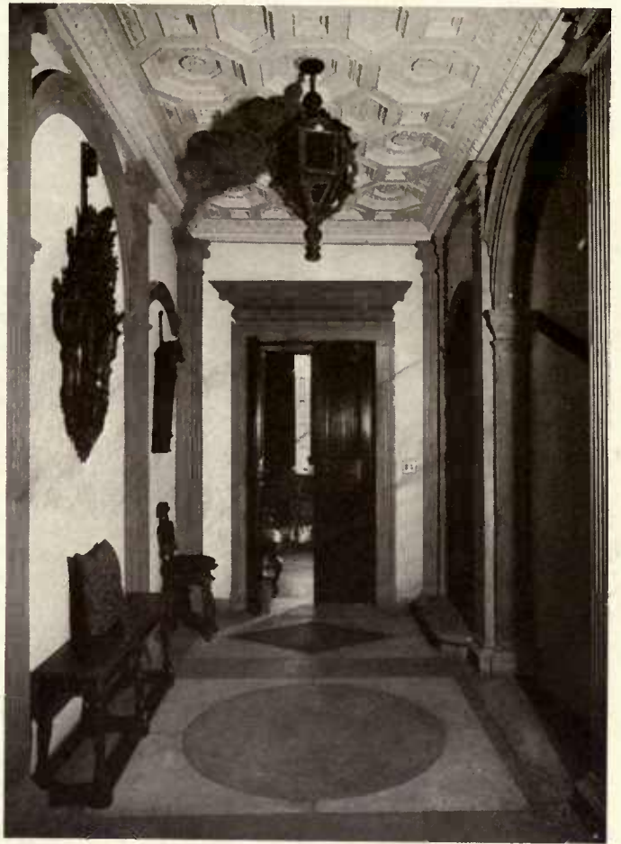
HALL, FIRST FLOOR.
