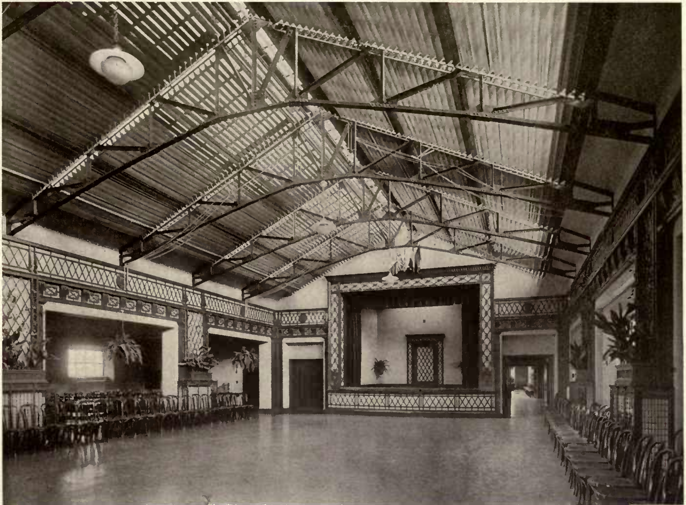
AUDITORIUM, SIXTH FLOOR.
