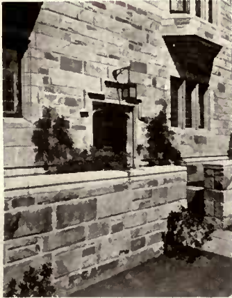
King Entry, Branford Court.
