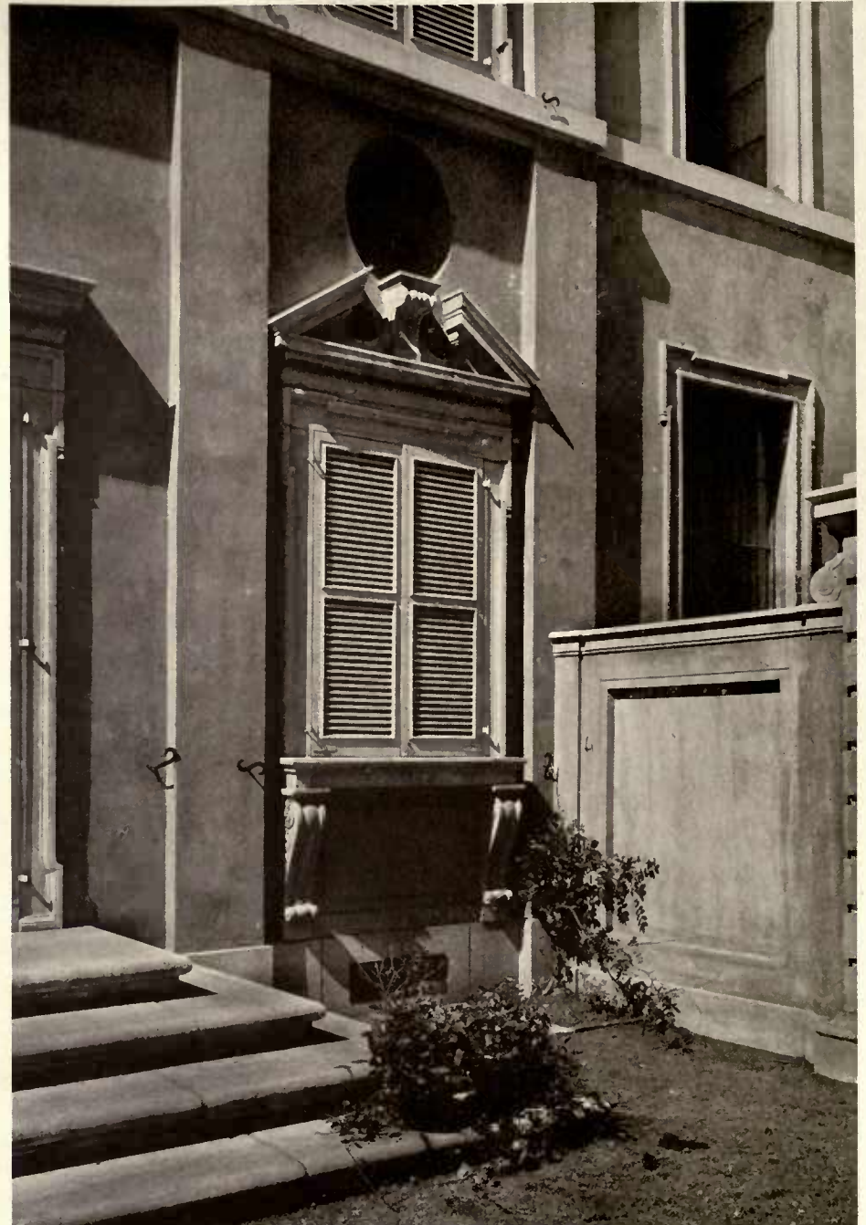
DETAIL OF DINING-ROOM WINDOW.
