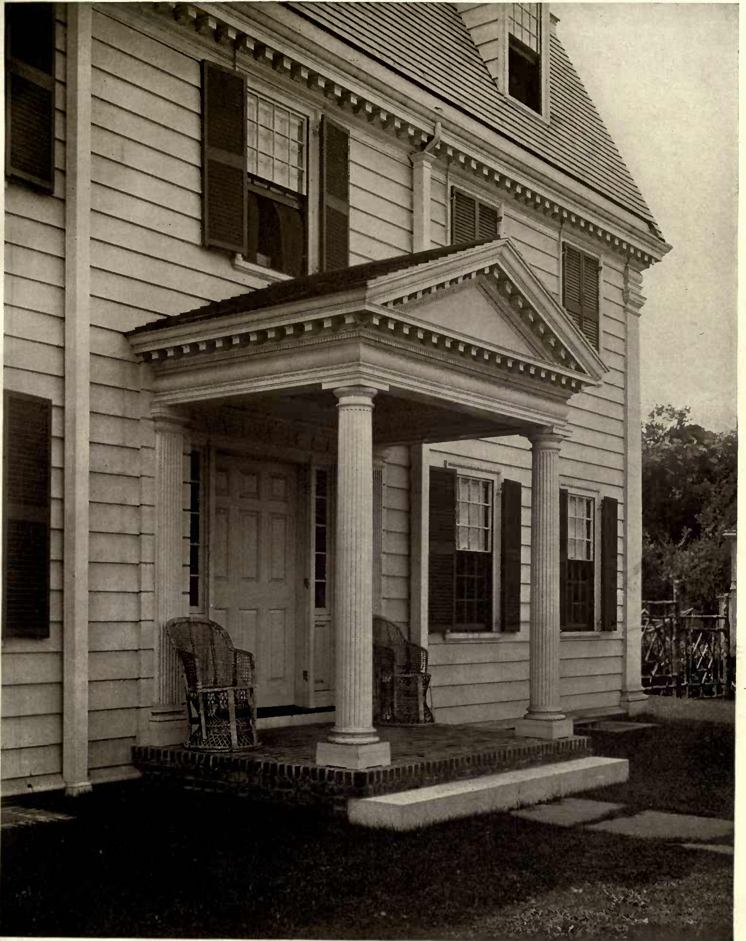
MAIN ENTRANCE, RESIDENCE, MRS. FRANK E. DODGE, STONINGTON, CONN.
