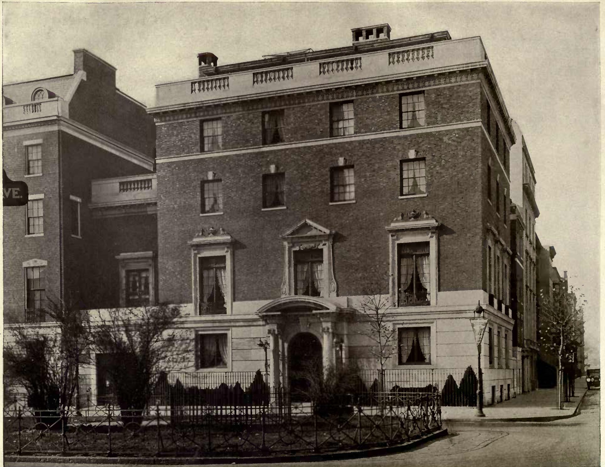
RESIDENCE, HENRY P. DAVISON, 690 PARK AVENUE, NEW YORK.
