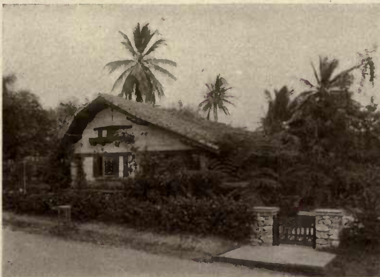
Architect's residence, Monte Flores, P. R. Reinforced concrete, old Spanish tile roof, mosaic floors, solid mahogany interior finish. Antonio Nichodema, Architect.
