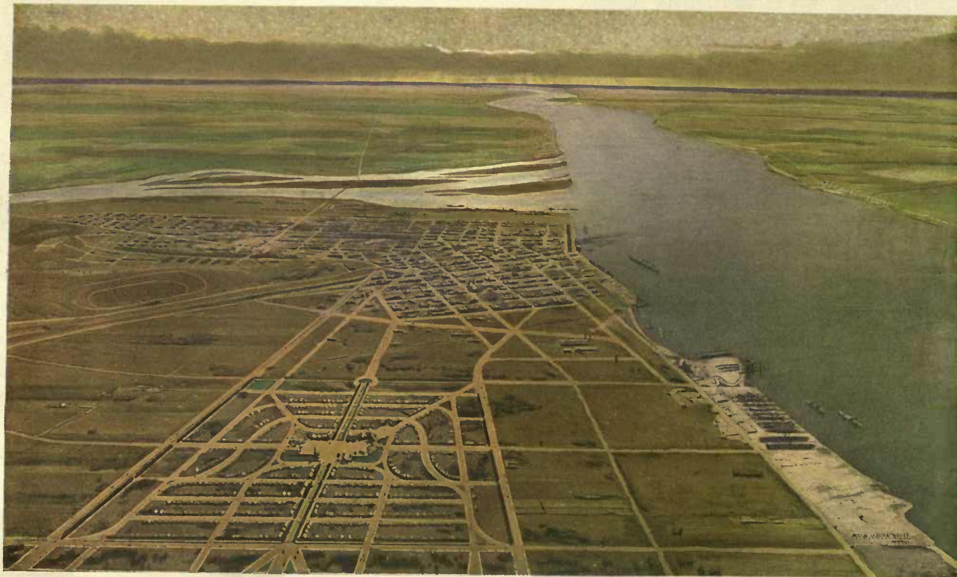
BIRD'S-EYE VIEW OF THE GREATER CITY OF THREE RIVERS, P. Q., CANADA, SHOWING NEW DEVELOPMENT IN THE FOREGROUND. Mann & MacNeille, Architects and Engineers.
