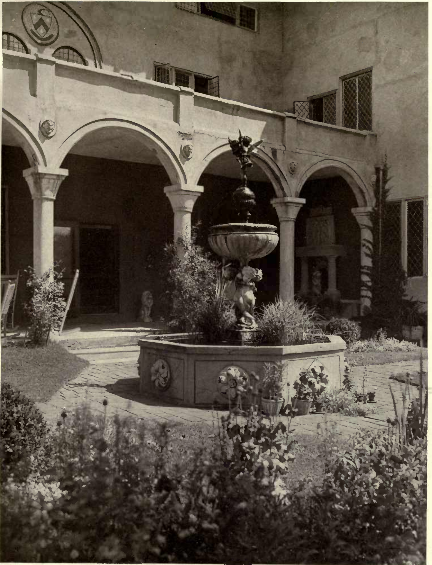
SOUTH PORCH, "TAMARACKS," RESIDENCE, FRANKLIN G. COLBY, ANDOVER, N. J.
