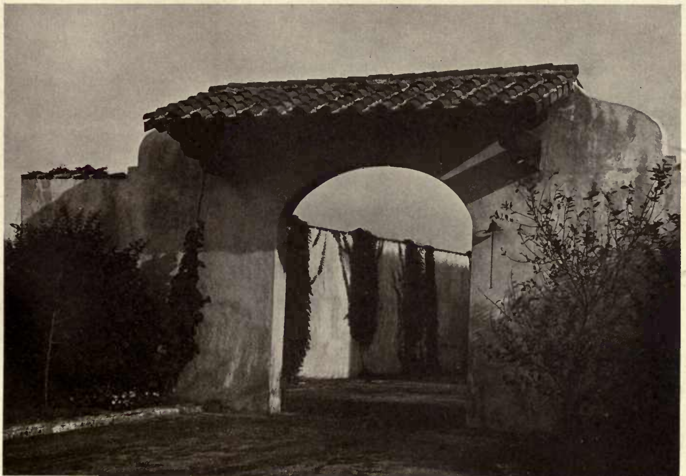
ENTRANCE TO SERVICE COURT.
