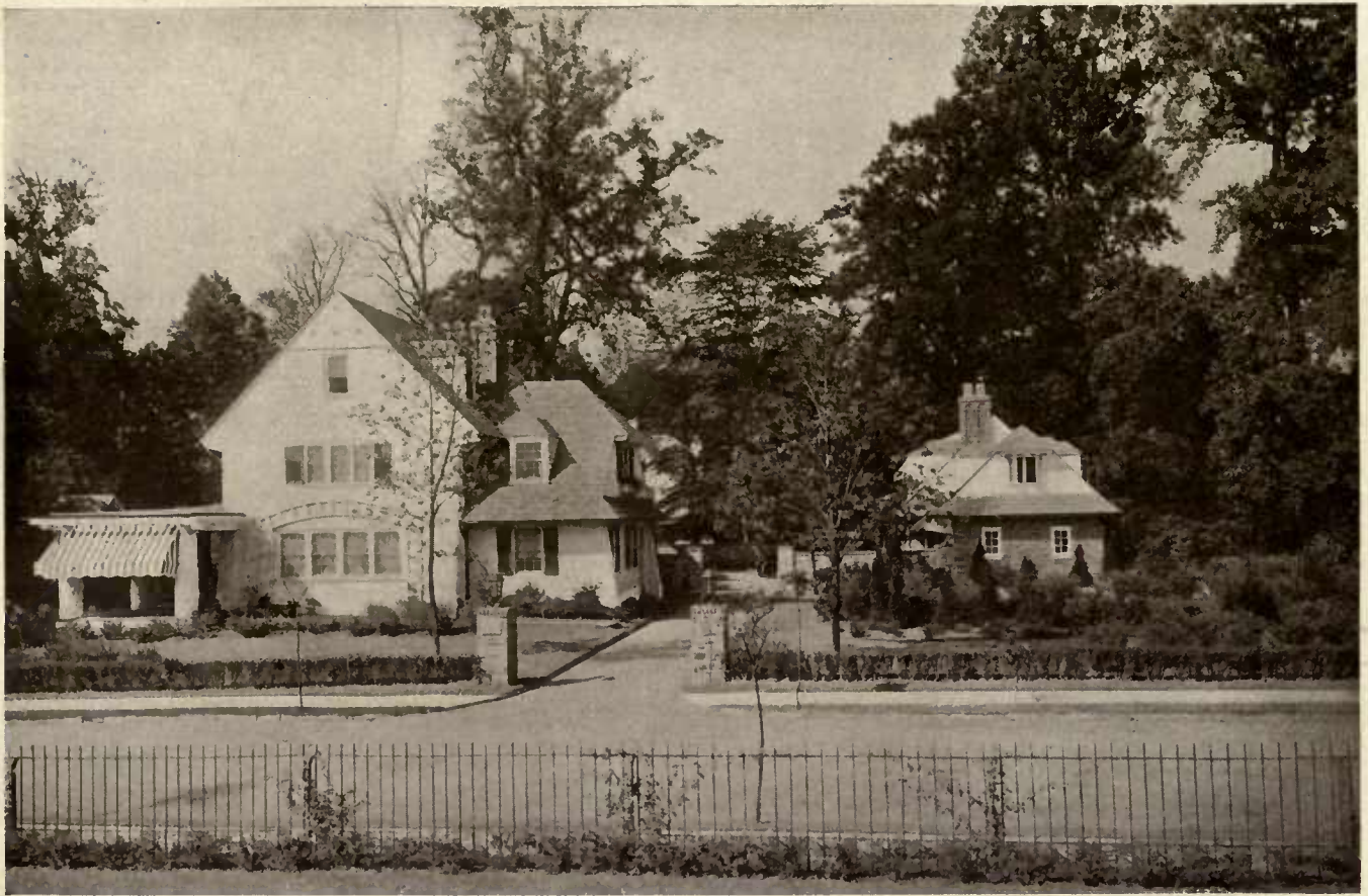
HOUSE AND GARAGE.
