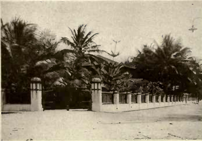
Fence for Ramon Valdes, San Juan, P. R., made in concrete and mahogany, leaded glass domes and panels for main posts, with inlaid mosaic panels.
