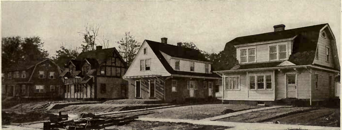
A group of recently completed houses in Firestone Park.
