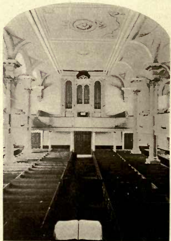
Interior, looking toward Beaver Street.
