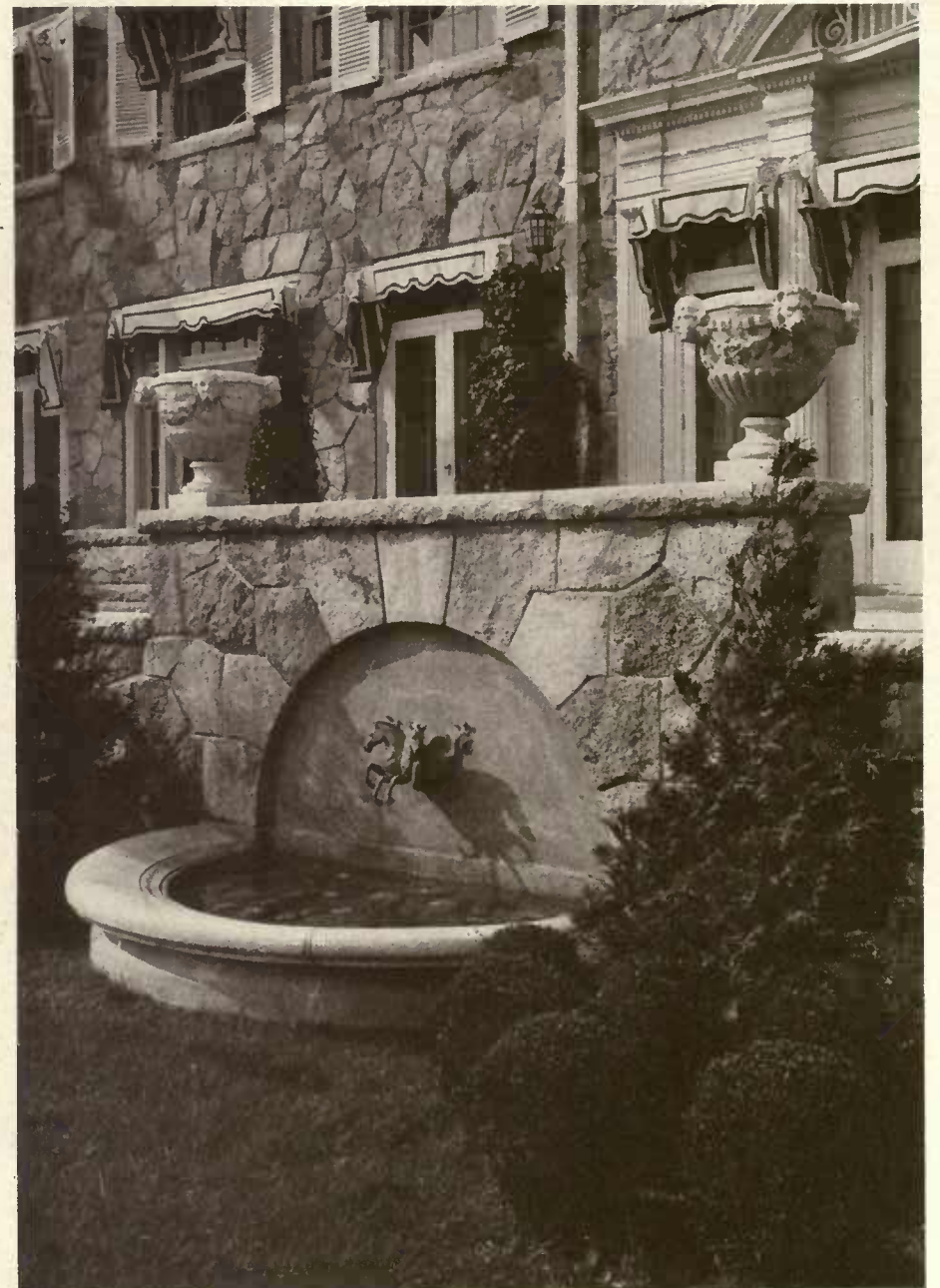
DETAIL ON TERRACE. Parker Morse Hooper, Architect; Frank C. Farley, Associated.
