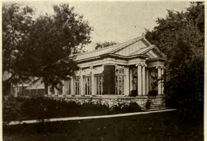
Conservatory and greenhouse attached to residence. W. P. Worth, Coatesville, Pa
