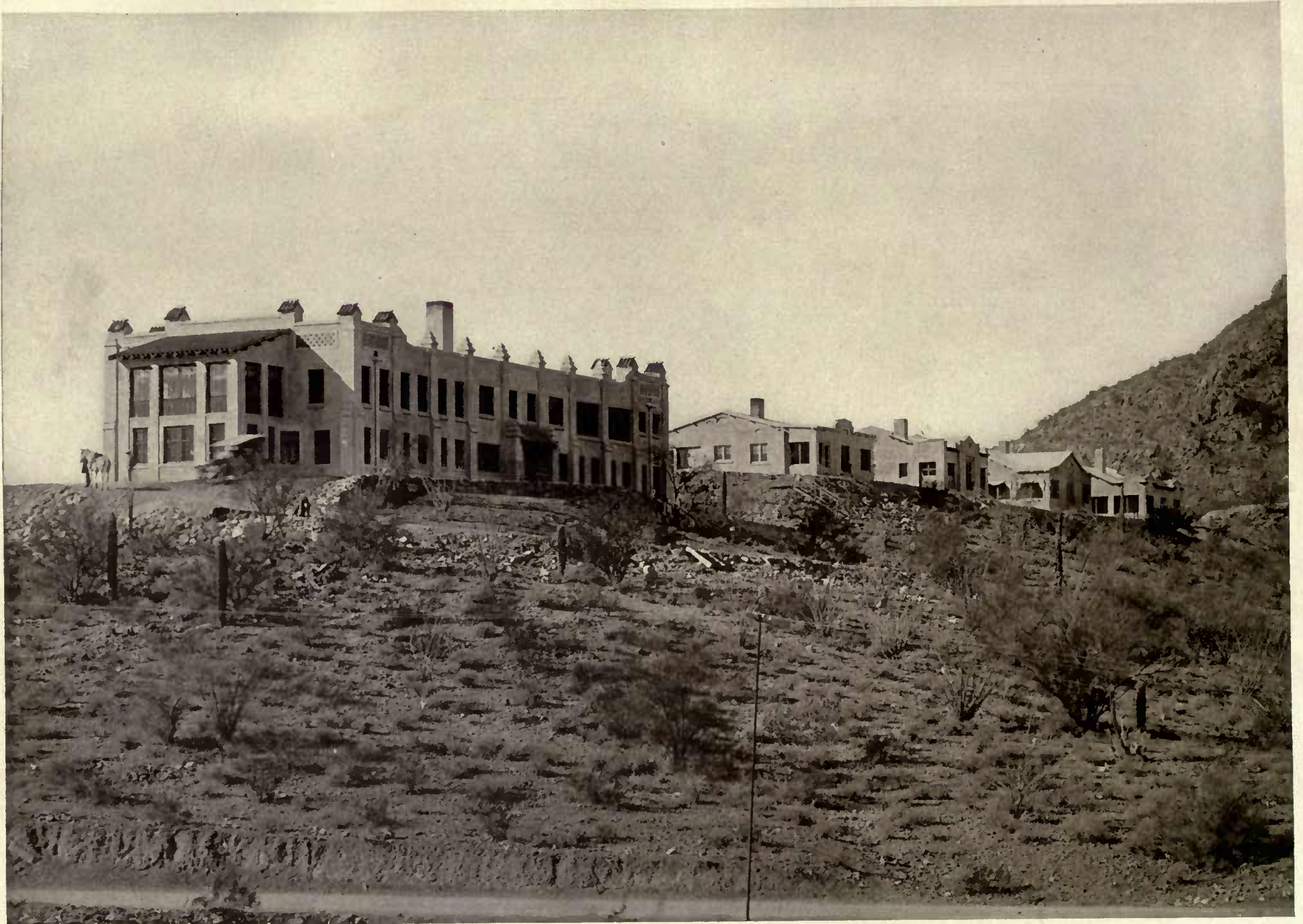
HOSPITAL WITH HOUSES, TOWN SITE, NEW CORNELIA COPPER CO., AJO, ARIZONA.
