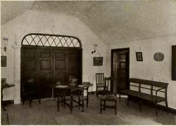
"Waterlot," Southampton; parlor, showing "tray" ceiling. Parge ornaments added c. 1770.
