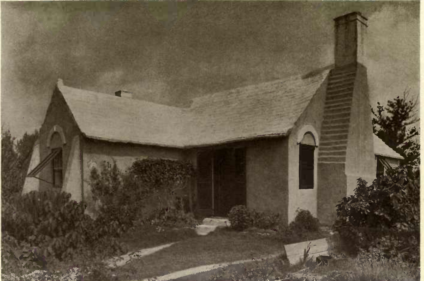
"St. John's Hill House," Pembroke; built c. 1690. Especially interesting as showing not only chimney base with battered weathering, drip-stones, and cruciform plan—this was adopted to secure all the circulation of air available—but also buttresses and ball finial at gable peak.
