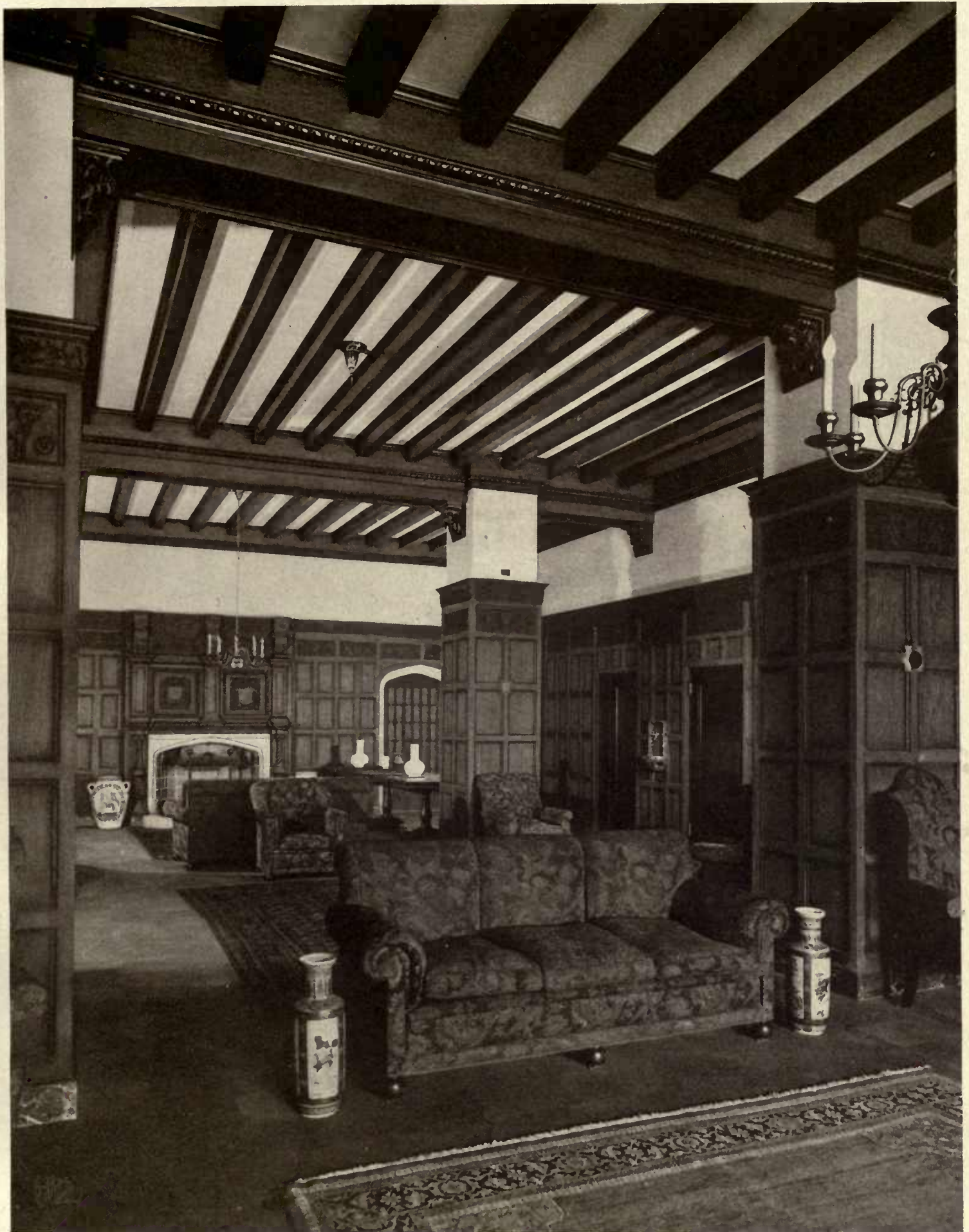
MERCHANTS' CLUB, BUSH TERMINAL SALES BUILDING, WEST 42D ST., NEW YORK.
