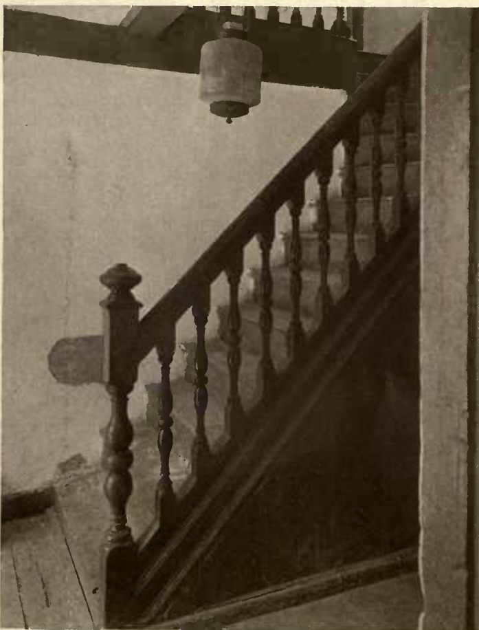
STAIRCASE DETAIL FROM LATE SEVENTEENTH CENTURY HOUSE IN ST. GEORGE'S, NOW OCCUPIED AS A NEGRO TENEMENT.
