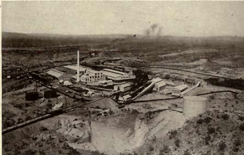
Ajo plant of New Cornelia Copper Company.
