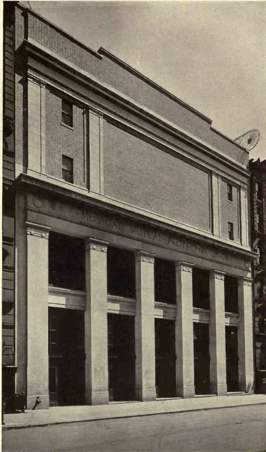
EAST 85TH STREET ADDITION.
