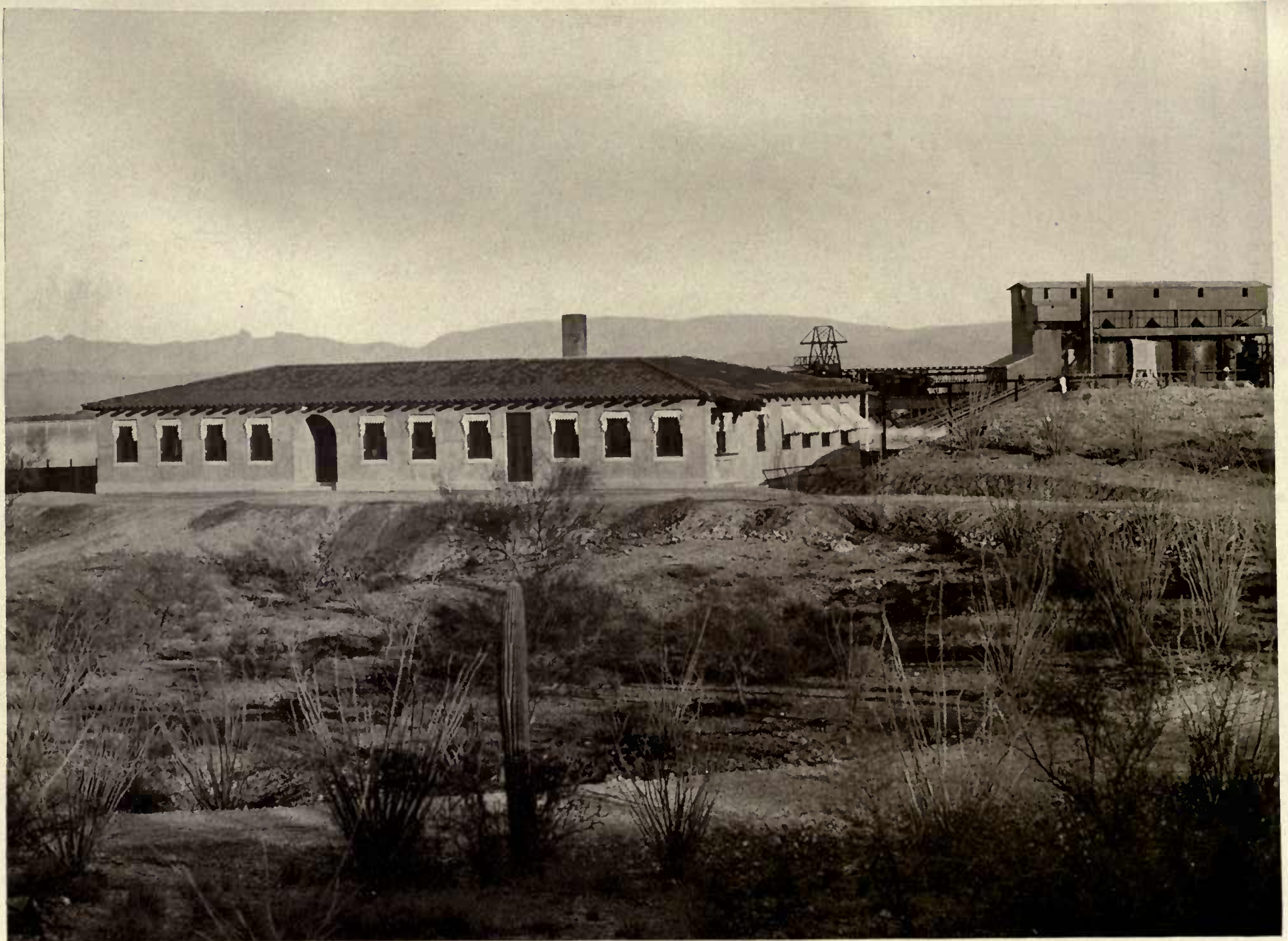
GENERAL OFFICE BUILDING, TOWN SITE, NEW CORNELIA COPPER CO., AJO, ARIZONA.
