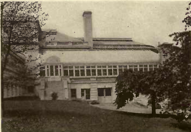
Side view of conservatory, residence, Capt. De Lamar.
