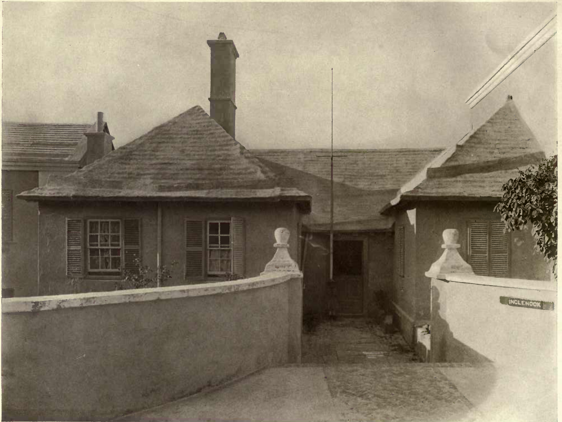
Early eighteenth century house, showing E plan, also ball finials of characteristic Bermuda contour on gate-posts.
