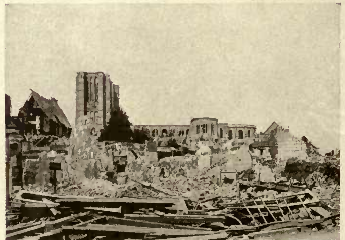
Cathedral of Noyon, June 1, 1919. The temporary roof is seen in place.
