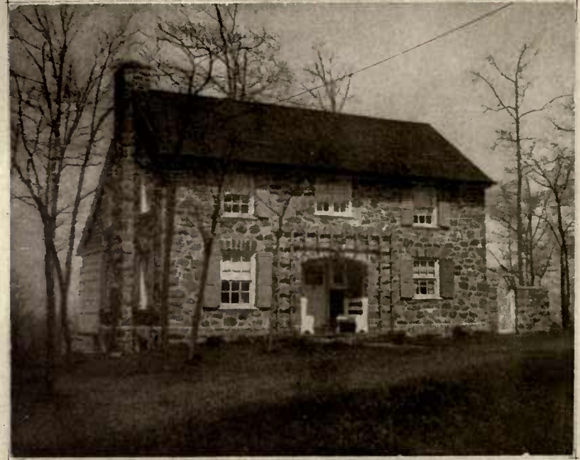
RESIDENCE AT ESSEX FIELDS, N. J. FOR E. LESLIE WINDENNY, ESQ. KENNETH W. DALZELL, ARCHITECT MAPLEWOOD, N. J.
