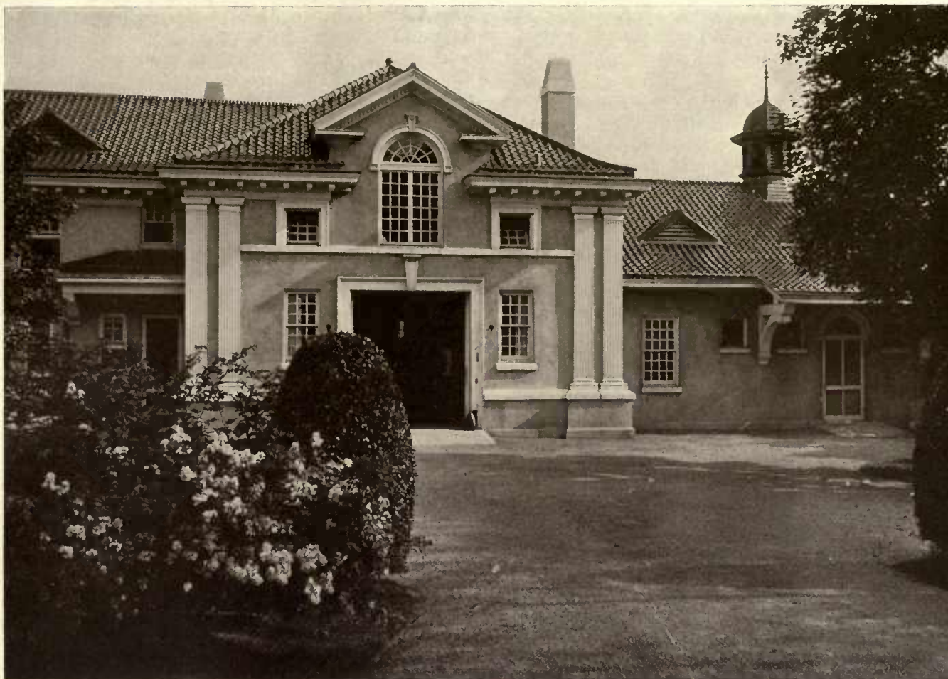
GARAGE, JOHN CHANDLER MOORE, OYSTER BAY, LONG ISLAND
