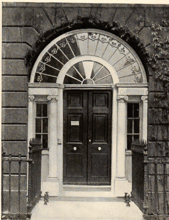
DOORWAY, 5 MANSFIELD ST
