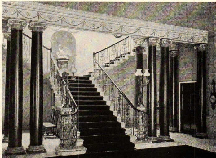
PRINCIPAL STAIRCASE, 1 PORTMAN SQ.
