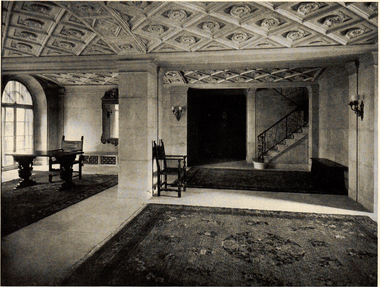
ENTRANCE HALL, ASTOR COURT APARTMENTS
