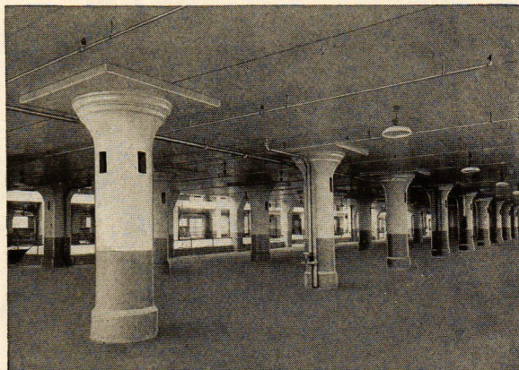
Column construction, showing air openings. Ford Motor Company's New Plant at Detroit. The heat for the system is from hot water pumped from the power house and circulated through VENTO Heaters. These are also used to cool the plant in hot weather, providing an average of 20 degrees cooler inside than outside temperature—83,000 sq. ft. of VENTO Heaters are in use in this up-to-the-minute factory.
