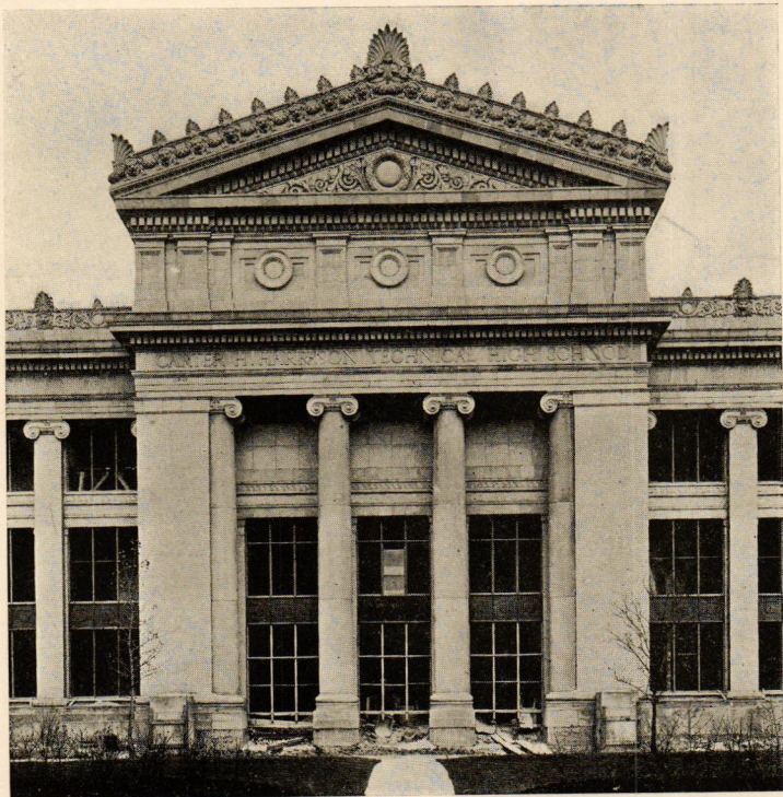
The Carter H. Harrison Technical High School, Chicago. A. F. Hussander, Architect.
