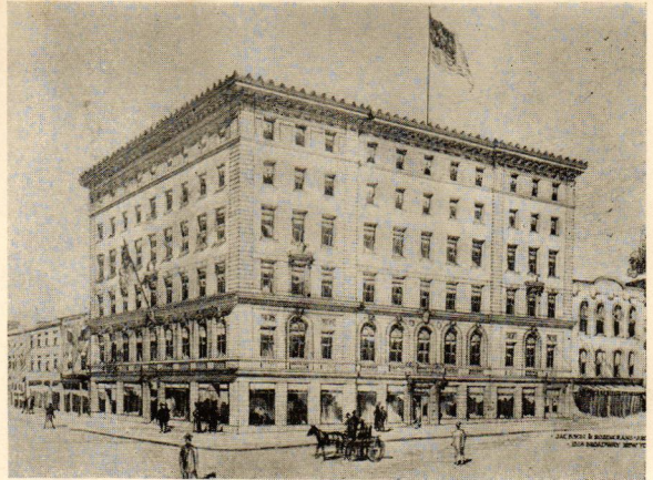
Y. M. C. A. BUILDING, WATERTOWN, N. Y. Jackson, Rosencrans & Waterbury, Architects.
