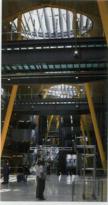
The undulated roof canopy at Terminal 4 is a complex assemblage of modular components (above left), supported by canted Y-form columns. Skylights admit daylight into the terminal interiors (above), which are crisscrossed by catwalks with glass pavers. Translucent ETFE louvers in the skylights help to distribute the daylight evenly through the space.
