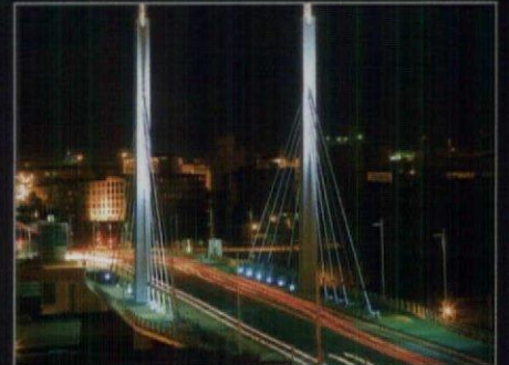
Sixth Street Bridge Milwaukee, WI
