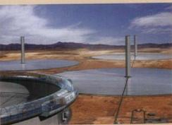
Morphosis' San Francisco Federal Office Building (left) forgoes mechanical air conditioning in 70 percent of the work area in favor of natural ventilation. In Schlaich Bergermann Solar's updraft tower (right), air is heated by solar radiation under a low circular translucent roof.
