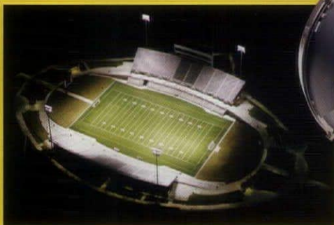
Sportsliter SG-V2 optics with maximum spill glare reduction minimizes light trespass around Round Rock Stadium in Texas.
