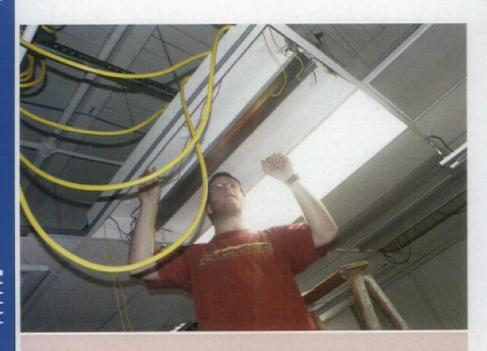
Students in the new lighting laboratory at Penn State University acquire hands-on experience with the benefits of DALI technology. Testing the functionality of a DALI control system involved retrofitting the standard electronic ballast used by the fixture with DALI-based ballasts.
