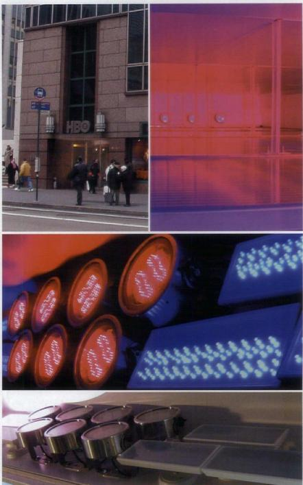
Television network HBO wanted to replace its understated black-painted glass panel signage (top left) with something more dynamic. Despite a very narrow space, lighting design firm Cooley Monato Studio created a vibrant sign using LED spots and wallwashers in waterproof housings (above and center), which light from the bottom up and provide color-changing capabilities. Four incandescent sources on a dimmer illuminate from the top down (top right).
