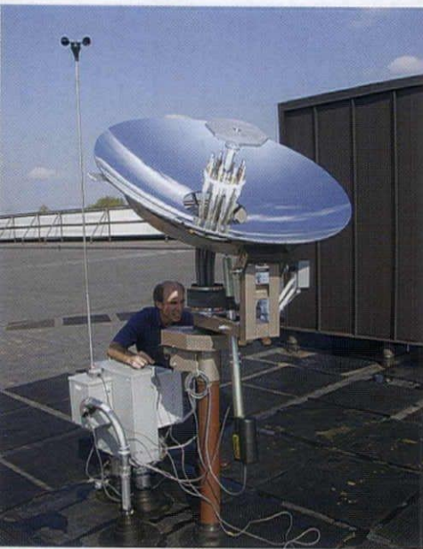
Hybrid lighting uses natural sunlight and electric light, as hybrid vehicles use both batteries and internal combustion engines. Roof-mounted collectors (above left) capture sunlight with flexible optical fibers and carry it into the building to special fixtures that also contain electric lamps. A control system keeps lighting levels constant by dimming electric lights when sunlight is bright, and turning them up as the sky darkens.
