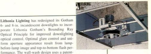
formance. The wall-wash design uses a patented hybrid polished kicker to provide uniform wall luminance with no back flash. An improved mechanical retention system ensures a secure fit for trims. Circle No. 141
