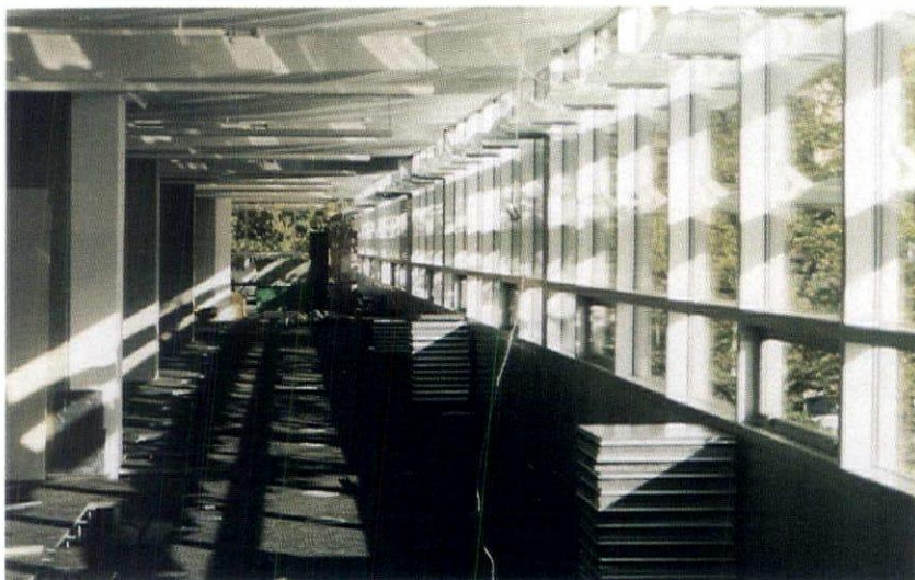
A common approach to bringing daylight indoors incorporates a light-shelf system into the architectural design. This facility in Canada utilizes curved glass to bounce light from exterior to interior.
