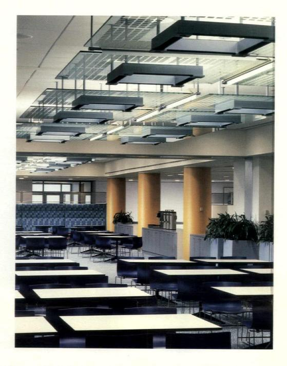
powerful light output. Metal halide downlights, recessed in the panels, add direct lighting. "When an entire room is indirectly lighted, things tend to flatten out," remarked Margulies. The square reflectors, radiused for the curved surface, add texture to the ceiling.
