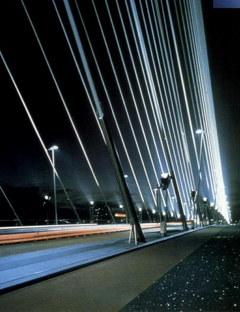
Above: Closer view of the pylon and cable lighting. The fixture structures, each with two or three projectors, can be seen along the bridge parapet. To avoid any glare, each of the lighting elements is mounted above the sightlines of all bridge users. In addition to providing the road and pedestrian lighting, the visible lighting columns also help illuminate the lower sections of the cable.
