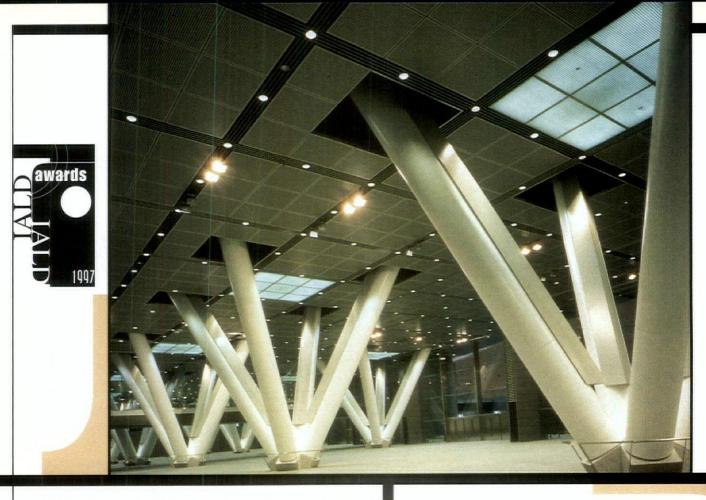
The lighting design for the subterranean exhibition hall (5,000 sq. meters) is also well equipped for diverse activities. Fluorescent lamps are attached at the top of the V-shaped columns, highlighting the structural design, while 150W metal halide downlights and incandescent track fixtures provide more lighting options within the open areas.
