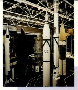
IN A RETROFIT OF A LARGE EXHIBITION GALLERY AT THE NATIONAL AIR AND SPACE MUSEUM IN WASHINGTON, D.C., THREE 90-FT.-LONG LIGHT PIPES, EACH CONNECTED TO A SULFUR LAMP, REPLACED 94 MERCURY VAPOR LAMPS, REDUCING ENERGY COSTS BY 25 PER-CENT WHILE INCREASING LIGHT LEVELS BY THREE TIMES.
