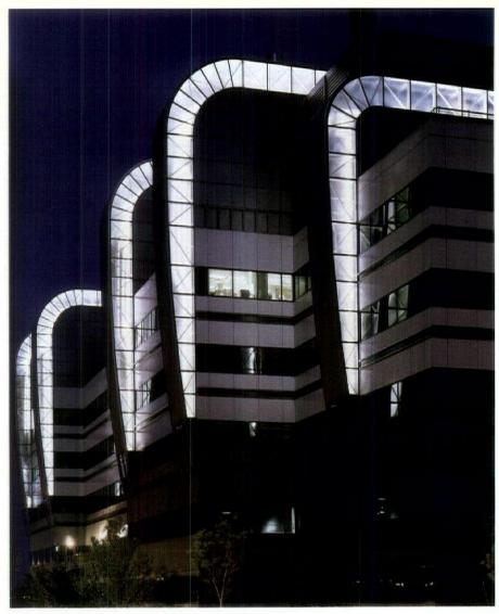
RIB-SHAPED INTERNAL SERVICE CHUTES ARE LIGHTED WITH FLUORESCENT SOURCES
