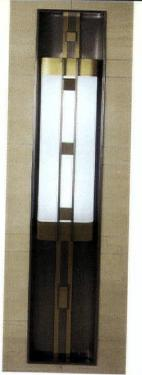
FILLING THE NICHE: The lighting fixtures in a lobby on Manhattan's upscale 57th street (far left) utilize vertical niches in the walls. Energy-efficient compact fluorescent lamps illuminate the recessed metal panels (left), creating both direct and indirect lighting.
