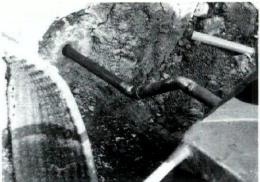
FOUNTAIN FIBER-ING: (Below) Ten black fiberoptic cables have been threaded through the central fountain sculpture. FAN POWER: (Above left) Cool air needed for the illuminators passes from one vault to the next through 6-inch conduits. COPPER CONDUIT: (Above right) Two 50-strand cables (two per illuminator) exit the vault through 2-inch copper conduit.
