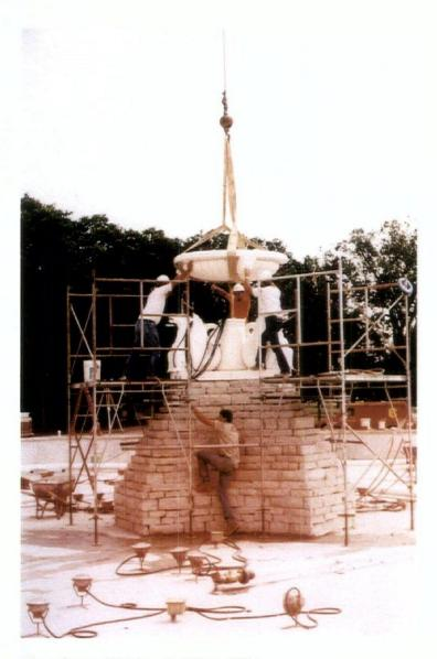
Corings allow water and fiberoptic cables into the sea horses, the lower bowl (six cables), the upper bowl (three cables) and one cable to the dolphin's mouth held by the cherub at the top.
