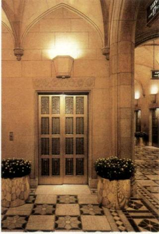
The Gothic ornamentation of the entry arch is illuminated by 90-watt halogen lamps, which are used as uplights behind the sconces. Cored into the bottom side of the wall sconces, 50-watt MR 16 recessed damp label fixtures are recessed and angled slightly inwards to create an asymmetric effect in each niche. One more 500-watt high-bay quartz downlight was added in the center of the entry's compound arched ceiling to brighten the floor and threshold.
