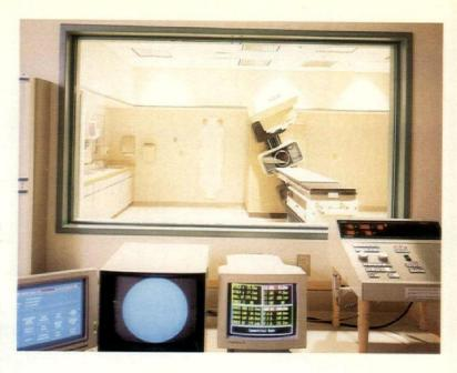
ers, and other technical equipment. The booth for the simulator area looks right into the room. But the booth for the therapy room is located behind 3 feet of solid concrete.
