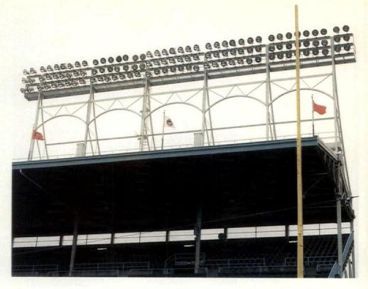
**OUT OF THE DARKNESS:** Sports floodlights have narrow beamspreads, as do these at Chicago's Wrigley Field. The maximum candlepower is contained within a beamspread between 18 to 70 degrees.
