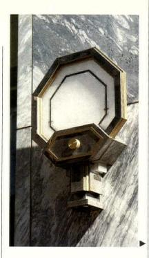
CHICAGO'S WATERTOWER PLACE EXTERIOR OCTAGON WALL SCONCE is manufactured by Appleton Lamplighter and designed by Green Hiltscher, Shapiro. The fixture measures 32 inches × 44 inches with a 9inch projection. The fixture is made of polished stainless and satin bronze, and the frosted lens is backlit with white neon. A 250-watt quartz lamp provides downlight. Appleton Lamplighter, Appleton, WI. CIRCLE 46.
