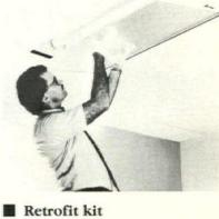
The Refractive Grid lens from Holophane is made to retrofit existing fluorescent fixtures; it reduces glare as much as 70 per-Because the lens decreases lumen output suited to locations where computers and VDTs are used. The lens fits into a nominal 2-by-4-foot exposed T ceiling grid with
