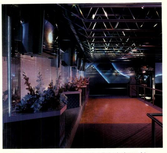
Above, PAR 36 pin beams aim colored light through this ceiling's painted trusswork in random directions to redistribute the dance floor's usual lion's share of light. At right, laser-etched diffractors produce fixed rainbow halations from PAR 46 pin beams that match the moving patterns produced by dual-scan units throughout the club.
