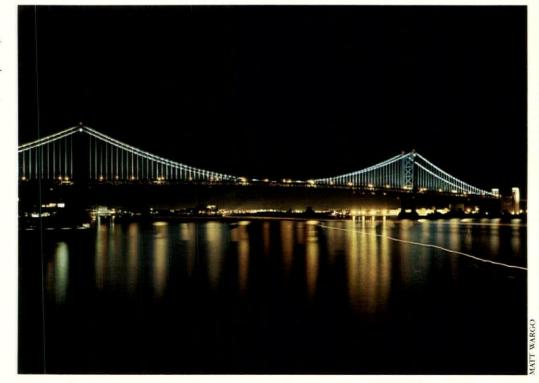
Award of Excellence winner. The lighting scheme for the Benjamin Franklin Bridge emphasizes the main catenary cables and vertical suspender cables that support the bridge deck. Computer-generated animation patterns are triggered by trains crossing the bridge.
