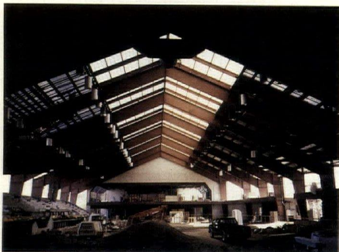
Translucent skylight panels prevent the harsh glare of direct sunlight without the use of blinds or shades. The glass fibers in the panels scatter light throughout the space and eliminate hot spots caused by direct sunlight.
