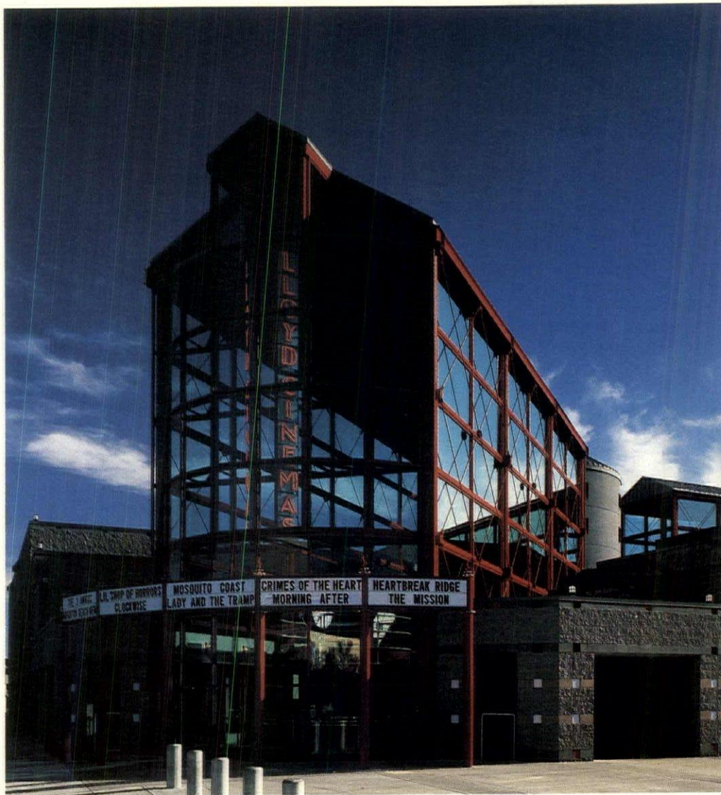
Roofs of the entry lobby, rotunda, and street of theaters soar above the lower roofs of 10 cinema houses.
