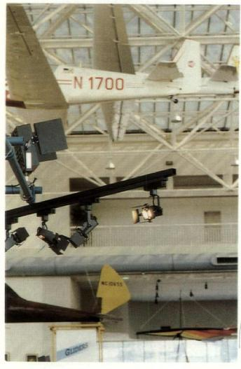
At night, photocontrolled 400-watt metal halide luminaires (top left) and ellipsoidal reflector fixtures (top right) wash the aircraft with light. Low-voltage track lighting (bottom left) illuminates interpretive displays.
