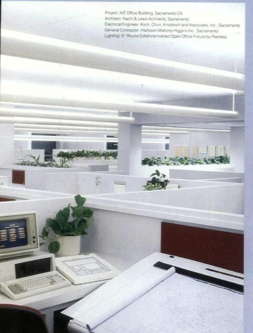
it. Any down light puts a bright light source in an unlit ceiling. The resulting strong contrast produces glare on any reflective surface: the cover of a magazine, a polished desk top or, unfortunately, a VDT screen.
