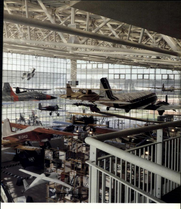
The triple-glazed reflective roof caused the highest heating and the lowest cooling loads; the Heat Mirror caused the opposite effect and admitted only a small amount of additional daylight. The triple-glazed reflective glass was eventually selected for use on the roof because the glazing would be installed in a nearly horizontal position. This would have caused stresses in the metal oxide–coated membrane of the Heat Mirror, and its long-term performance could not be guaranteed.
