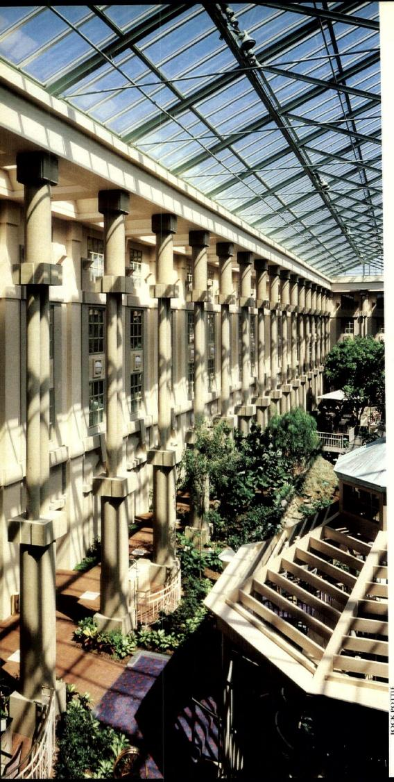
size, and orientation of the side walls and the percentage glazed affect the amount of light reflected into the atrium as well as the amount of heat absorbed by the walls and the amount of glare users of the atrium would experience. Every option had some bearing on the final cost of construction and future energy consumption.
